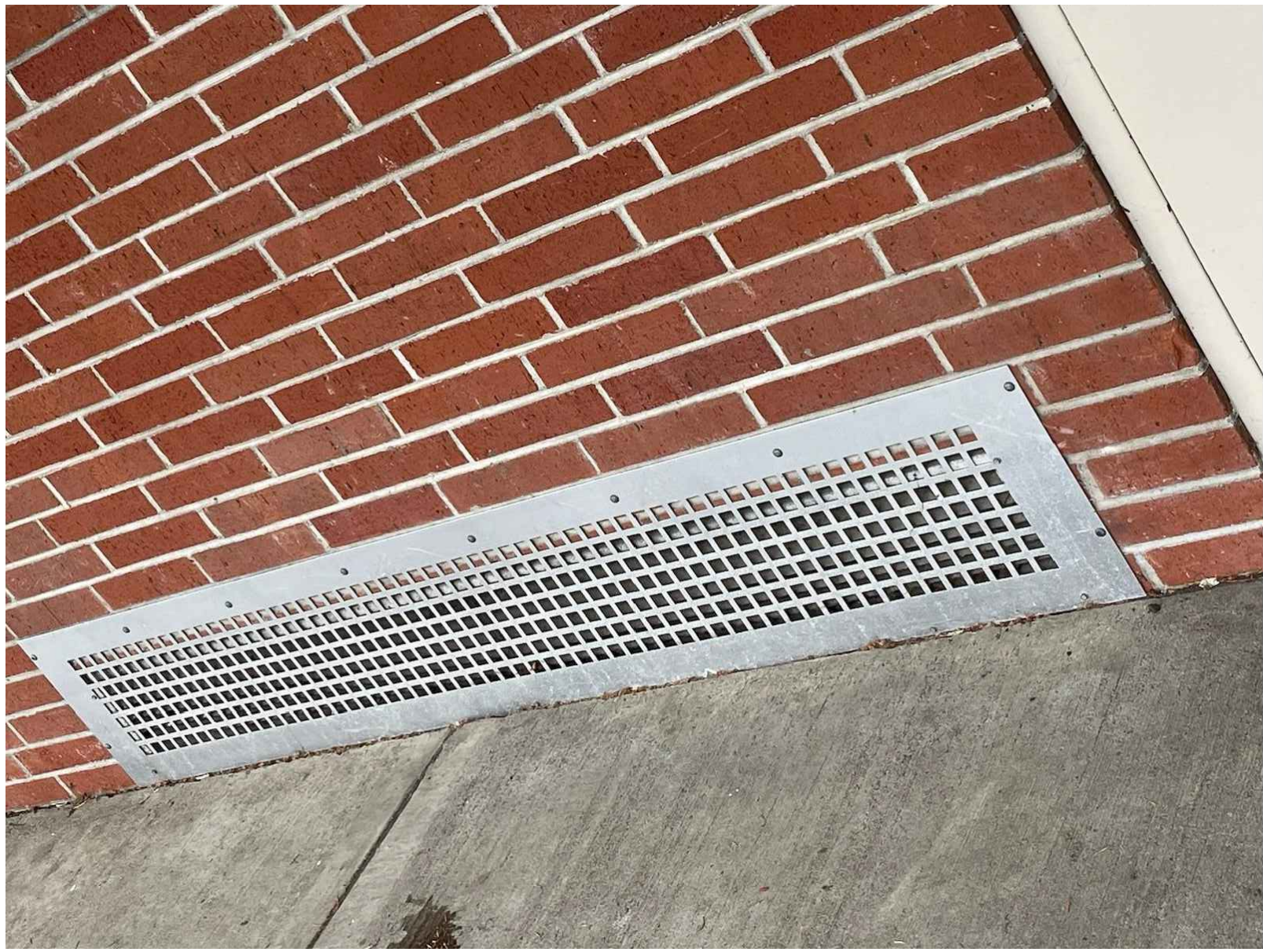
EXISTING VENTILATOR LOUVER
