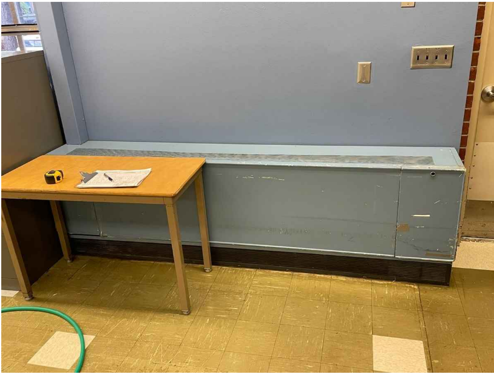
EXISTING UNIT VENTILATOR
