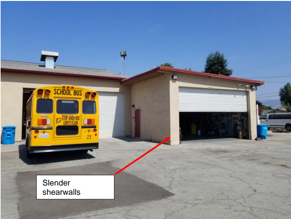
Figure 8 – Building 100 eastern shearwalls
