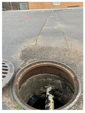
Photograph No. 12: Catch basin with sediment around structure. Note previous sawcut patch south of B-6, in east/west direction.
