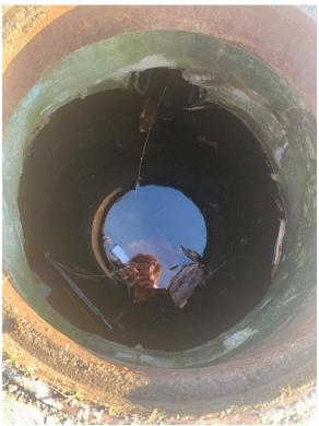
Photograph No. 15: Interior of precast storm structure with standing water.
