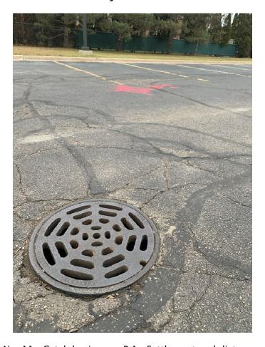
Photograph No. 11: Catch basin near B-1. Settlement and distress around basin.
