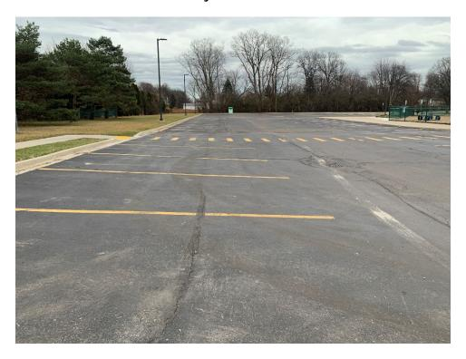
Photograph No. 13: Pavement west of areas to be reconstructed. Note settlement around drainage structure.
