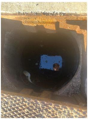
Photograph No. 19: Interior of precast drainage structure near B-2, holding water.
