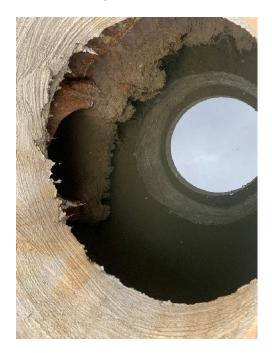
Photograph No. 18: Catch basin with newer concrete collar.
