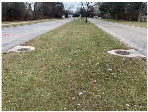
Photograph No. 18: Catch basins along interior of boulevard. Note newer concrete collars.
