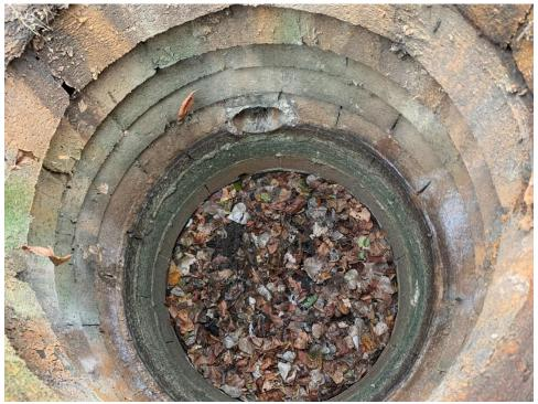
Photograph No. 17: Interior of catch basin adjacent to drain.
