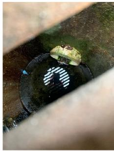
Photograph No. 17: Interior of precast structure with standing water.
