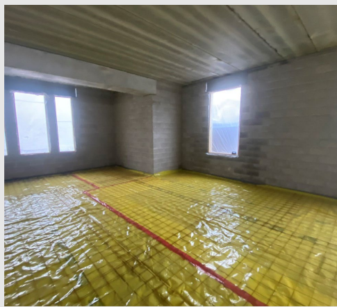
Pouring the concrete slab in the cafeteria and commons expansion is a process that includes installing the vapor barrier and reinforced steel mesh, letting the concrete cure, and then installing the control joints, which avoid cracking in the concrete
