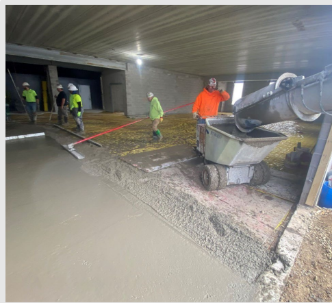
Pouring the concrete slab in the cafeteria and commons expansion is a process that includes installing the vapor barrier and reinforced steel mesh, letting the concrete cure, and then installing the control joints, which avoid cracking in the concrete
