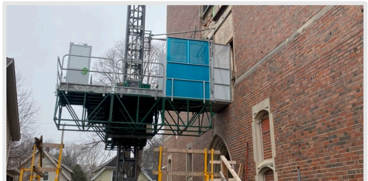
A temporary hoist with a carrying capacity of 3.2 tons was used on the west side of the building to bring construction materials in and out of the newly renovated classrooms
