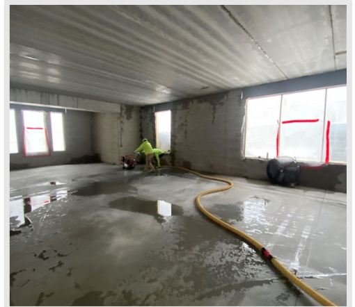
Pouring the concrete slab in the cafeteria and commons expansion is a process that includes installing the vapor barrier and reinforced steel mesh, letting the concrete cure, and then installing the control joints, which avoid cracking in the concrete
