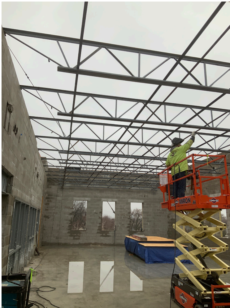
VEL PHILLIPS MIDDLE SCHOOL PLACING JOISTS AT THIRD FLOOR
