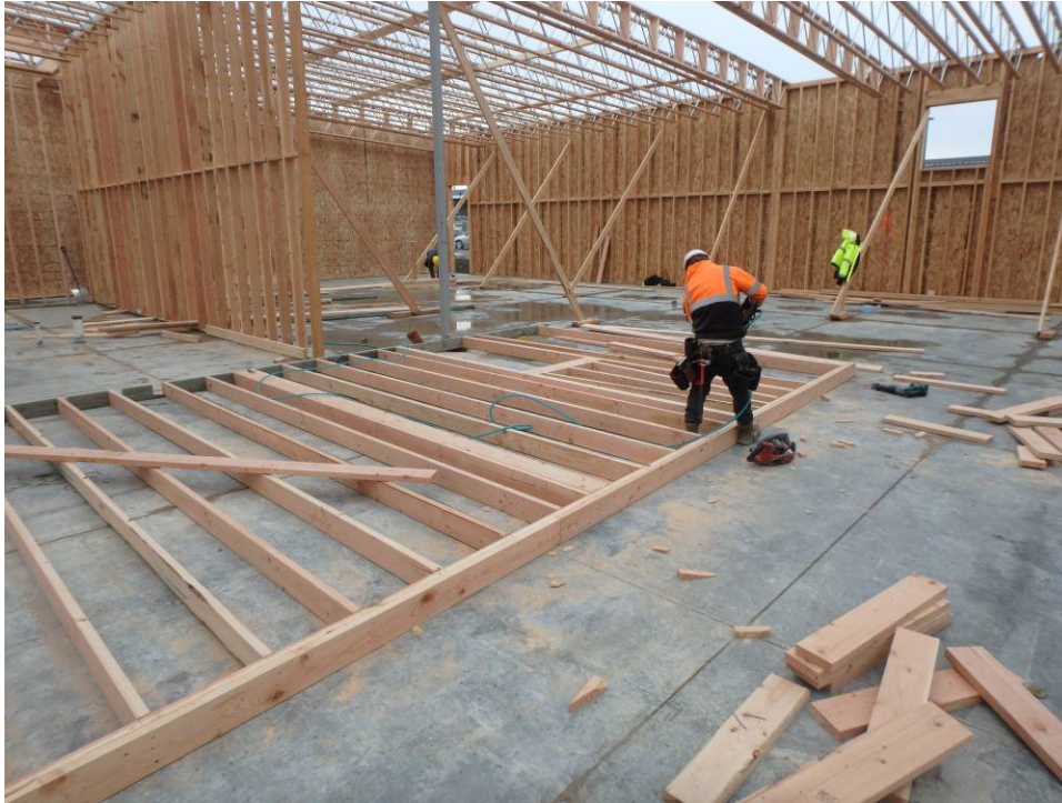
Framing interior wall
