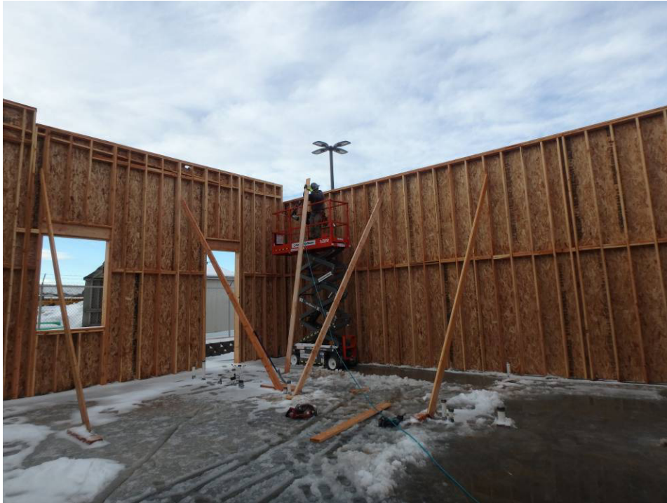
Setting the top plate and preparing for the new roof trusses
