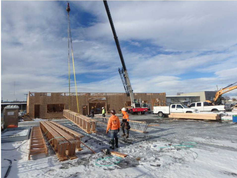
Picking the truss
