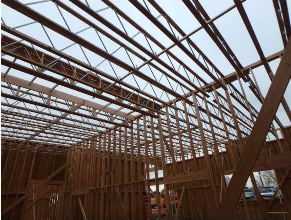
Looking northeast at the central east-west wall, all trusses are set
