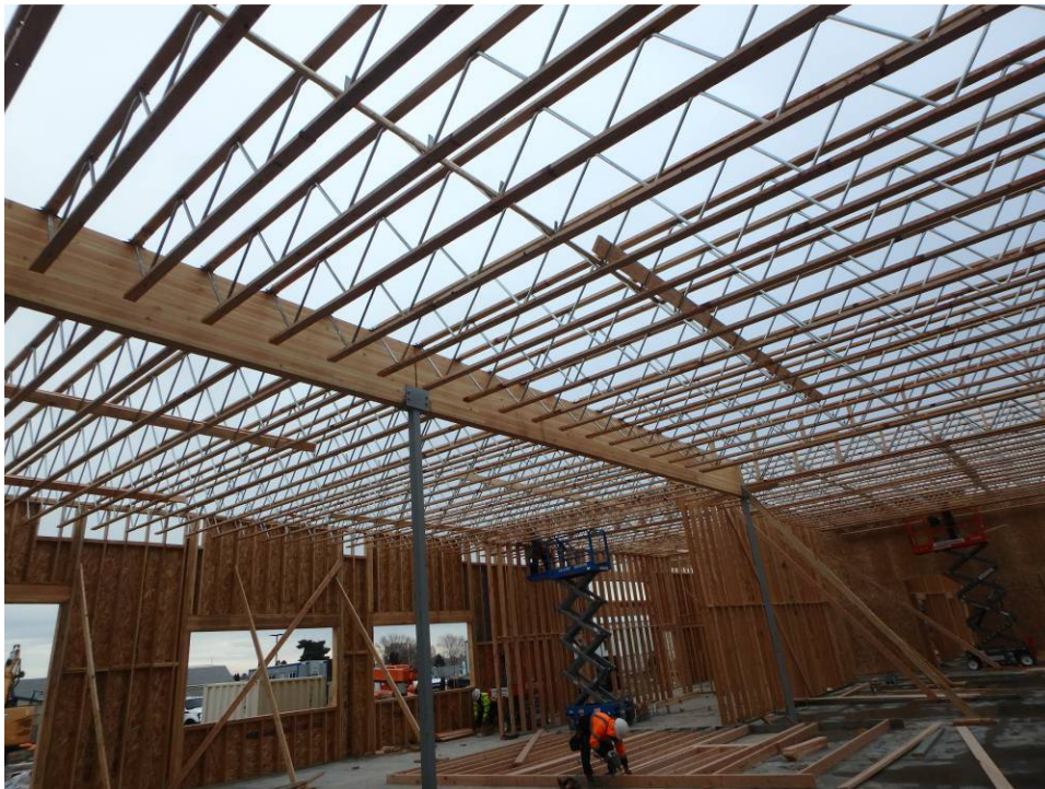
Looking southeast at the set trusses
