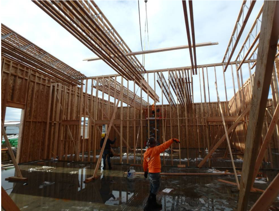
Crane - Moving trusses to the building
