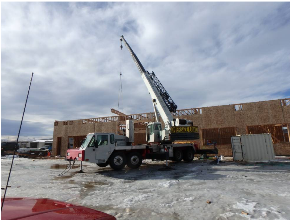
Crane - Moving trusses to the building
