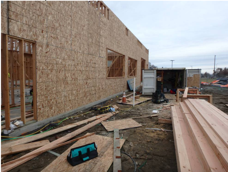
Looking north at the east wall framing and sheathing
