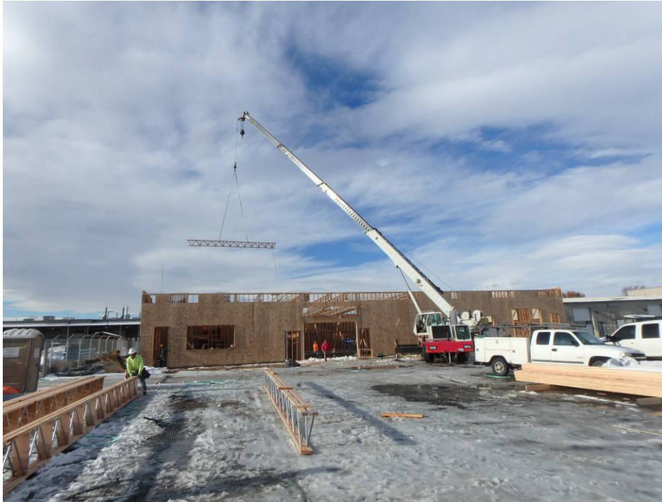
Moving trusses to the building
