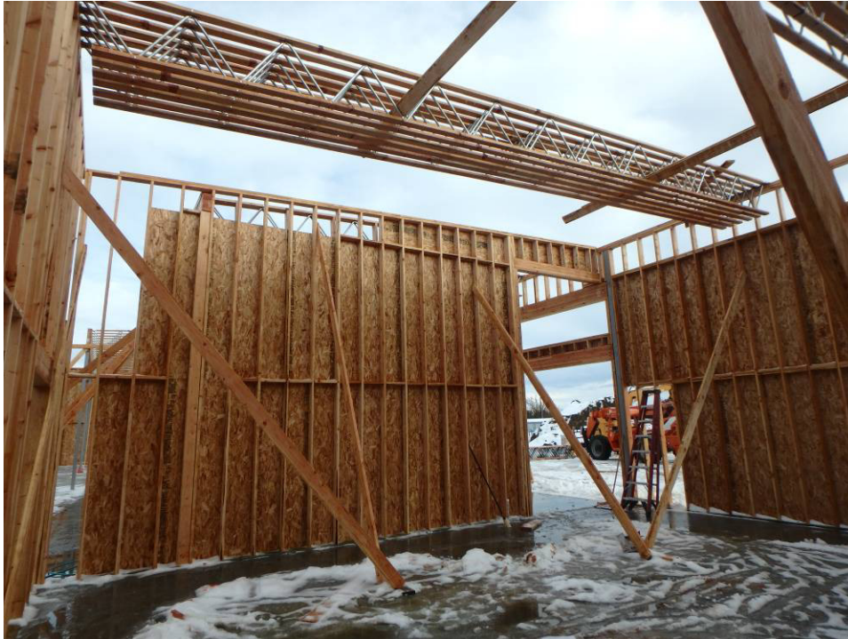
New roof trusses and central east-west wall framing
