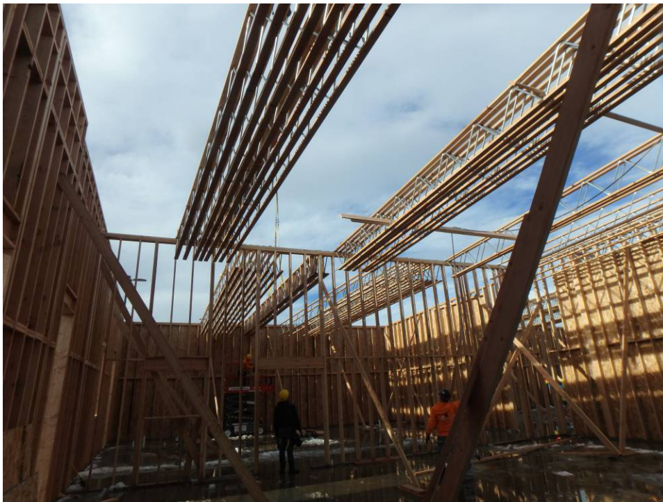
Trusses set on the south half of the building
