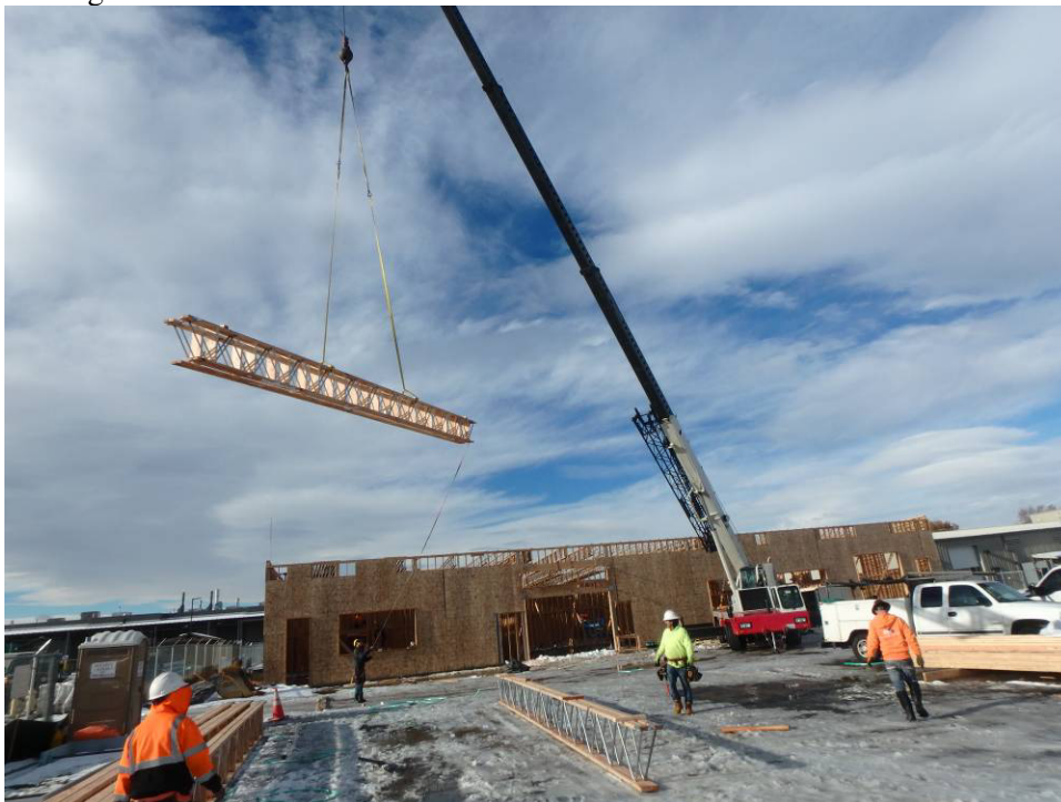
Moving trusses to the building
