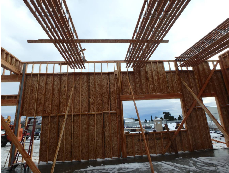
Looking at the east wall framing and the set roof trusses
