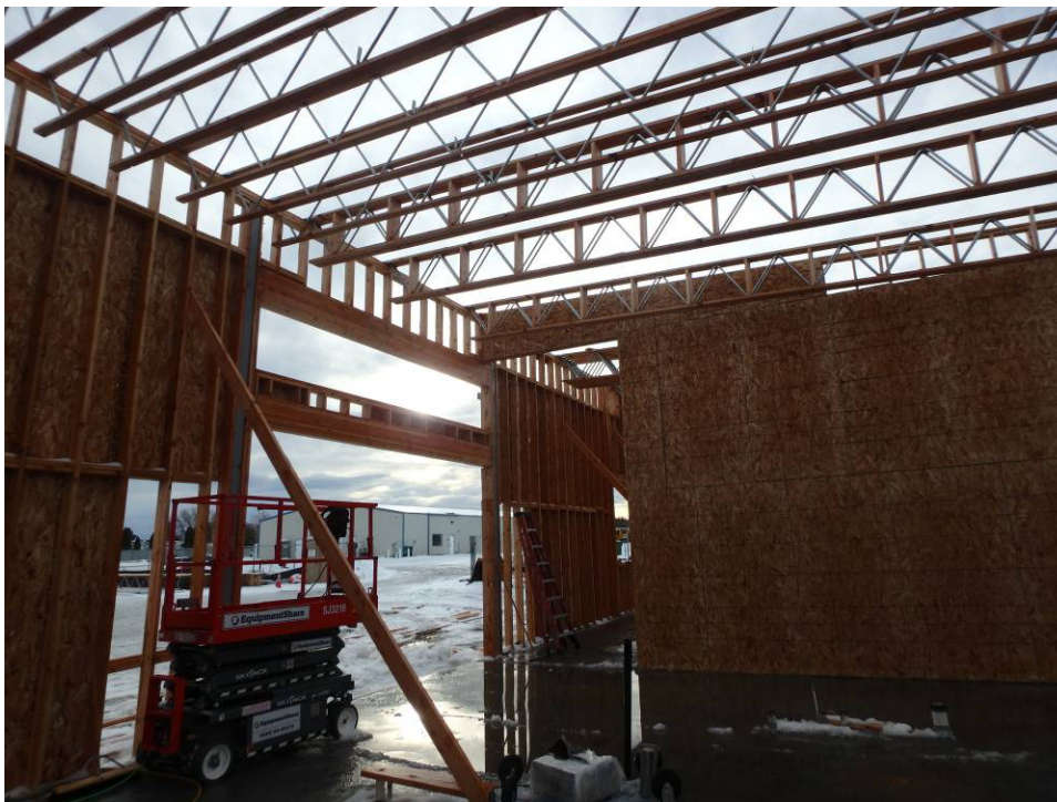
Trusses over the east wall central area
