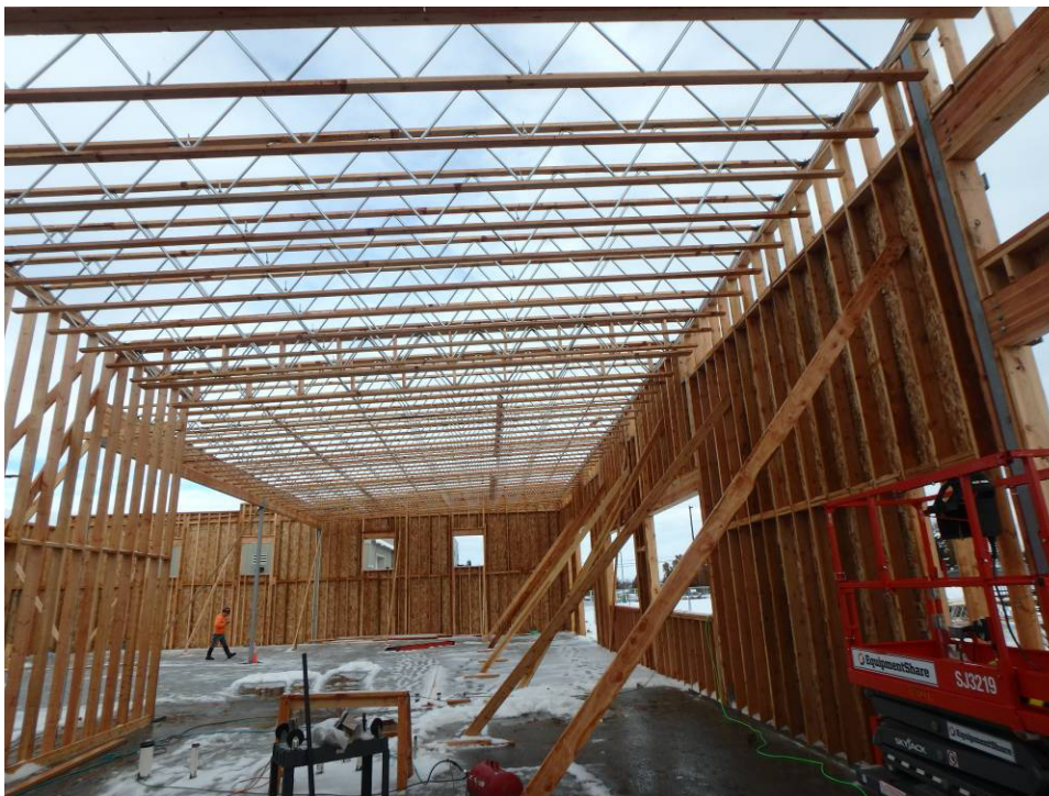
Northeast quarter roof trusses set
