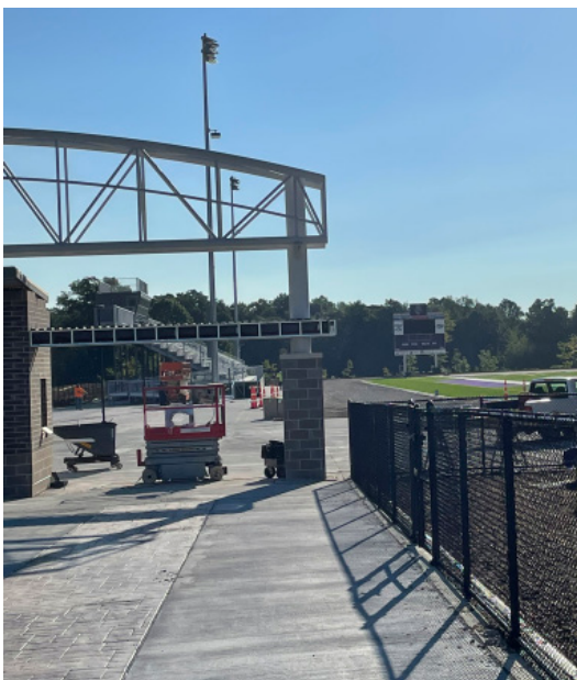
The new football field while under construction
