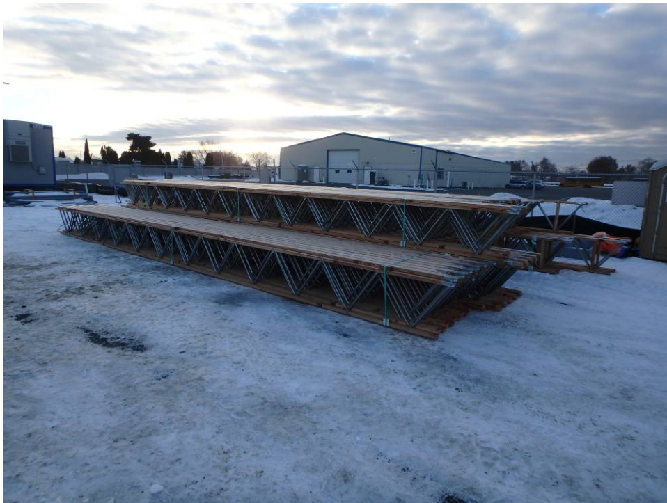
New roof trusses
