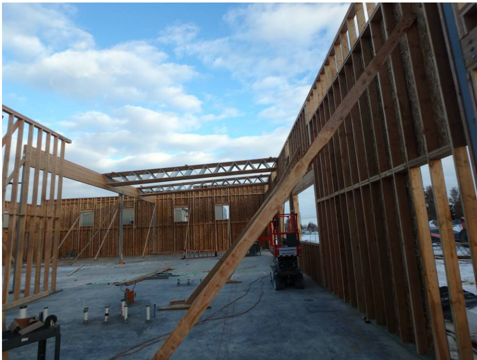
Looking at the East wall north framing, sheathing and set trusses
