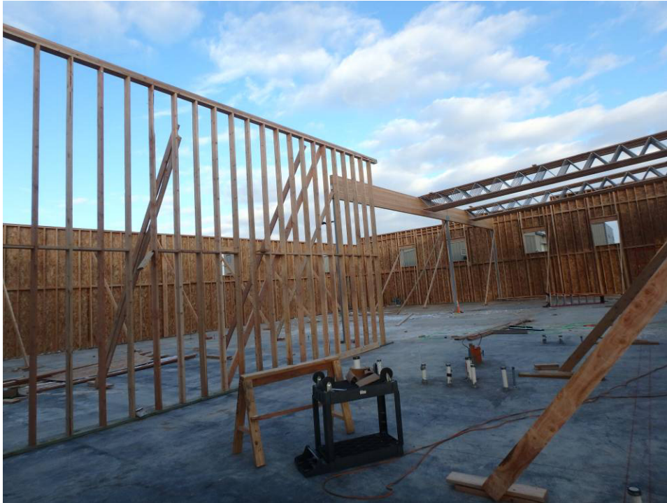
Looking northwest at the central wall and set trusses
