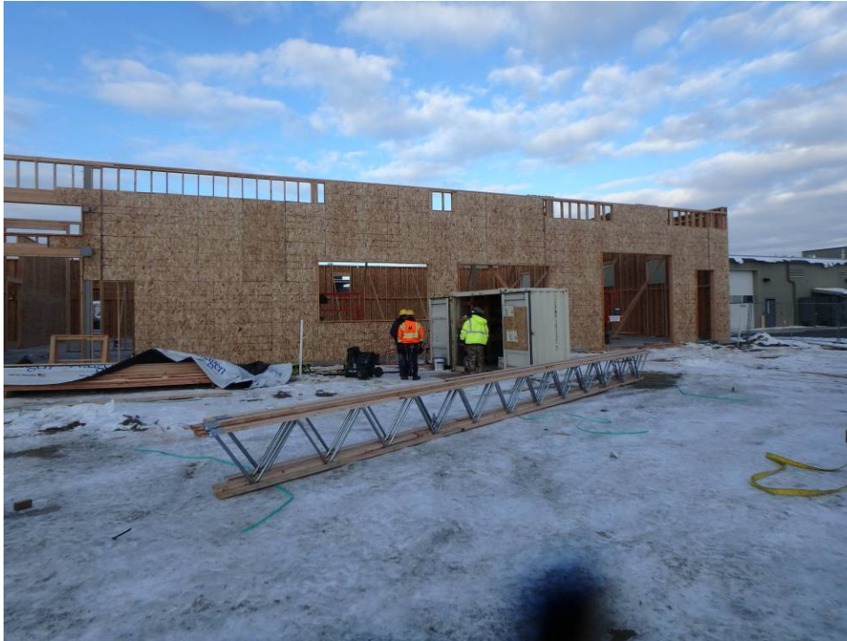
Looking at the east wall framing and sheathing
