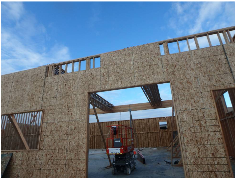
Looking at east overhead door wall framing and sheathing
