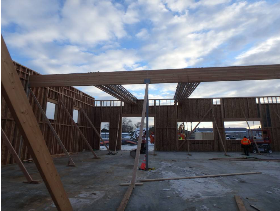
Looking east at the glue lam beam and trusses
