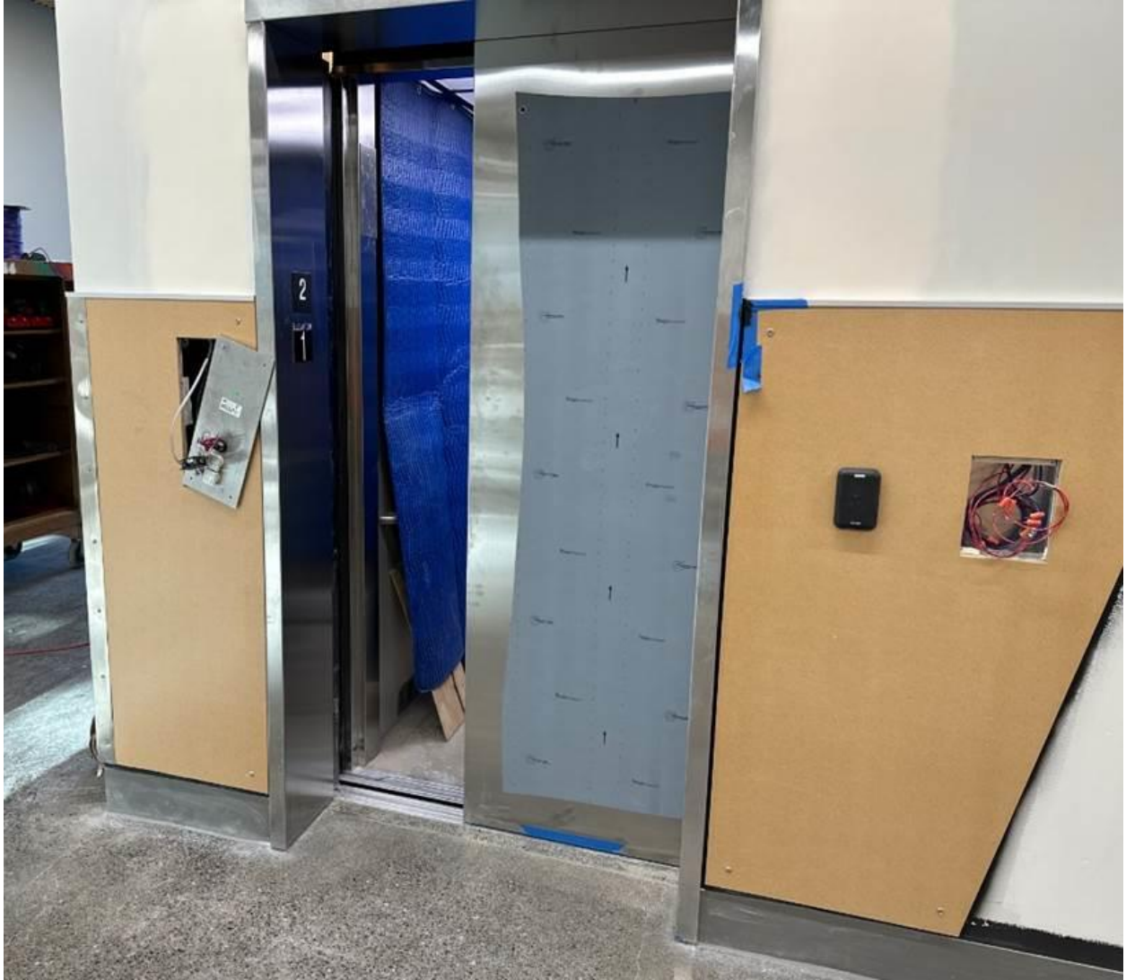
Final connections and elevator testing were completed this week
