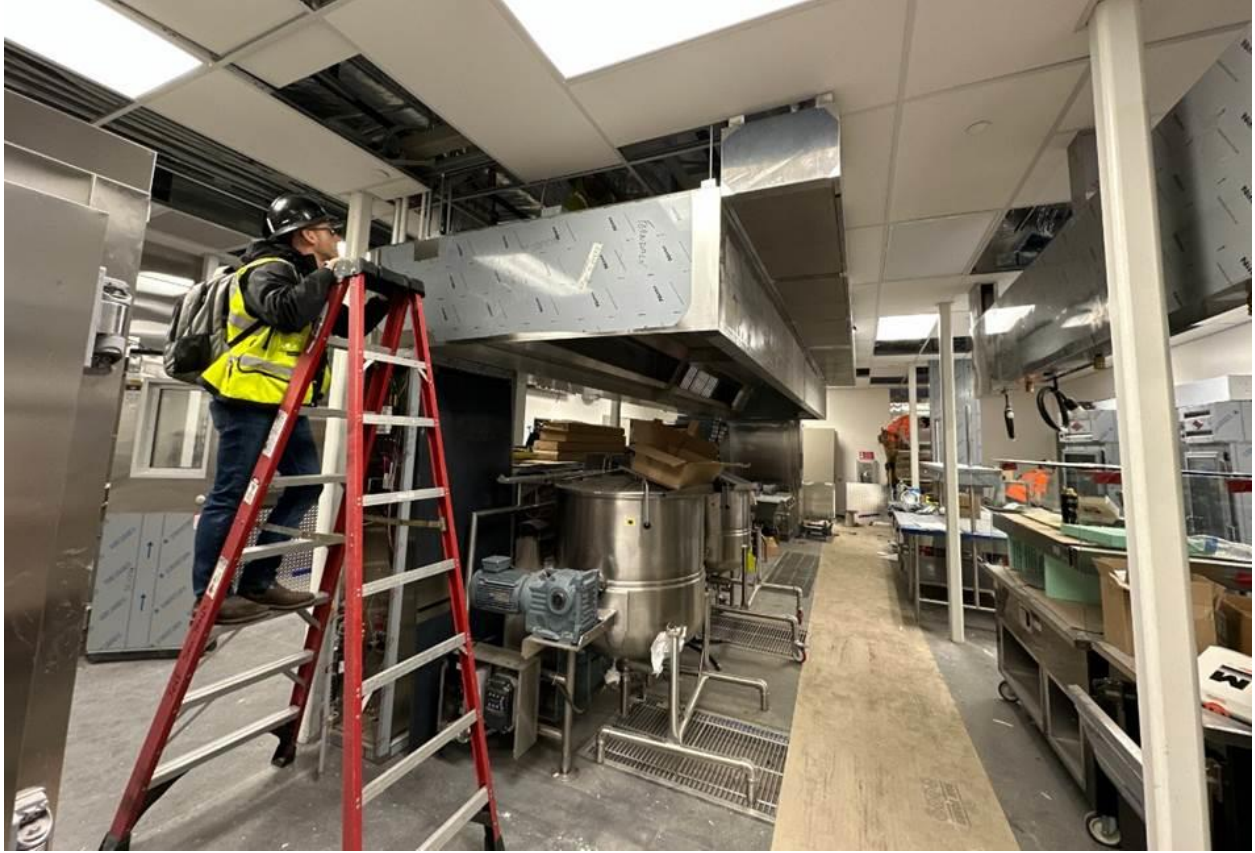
Final installation of the cooking line equipment in the kitchen
