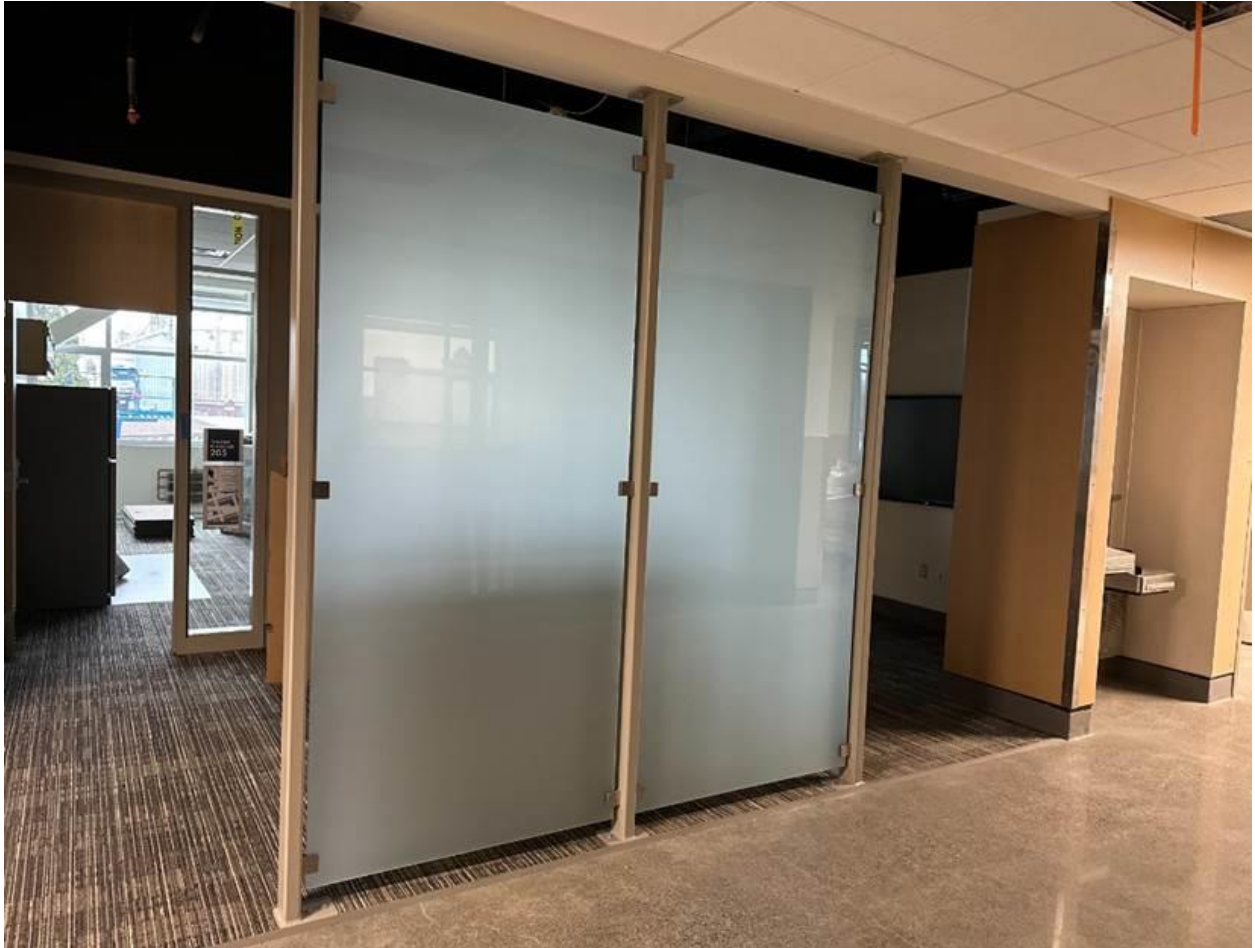
Final glass installation on one of the collaboration spaces
