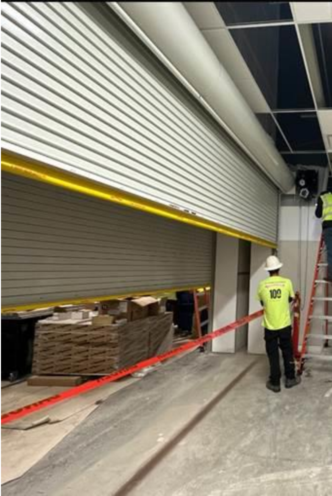
Final fire door testing occurred this week
