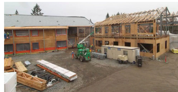
Mountlake Terrace Elementary construction site.
