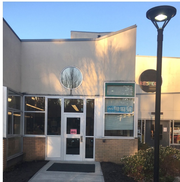
The new entrance (above) at Terrace Park Elementary controls access during school hours and entry is directly into the main office. The former main entrance can be seen to the right of the new entrance.
