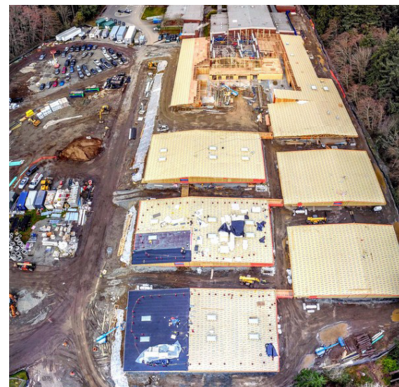
Aerial view of Madrona K-8 site.
