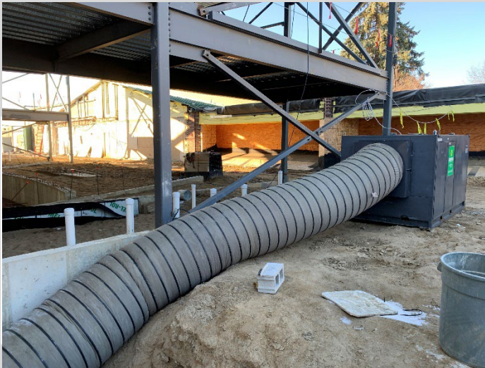
Temporary Heating Units
