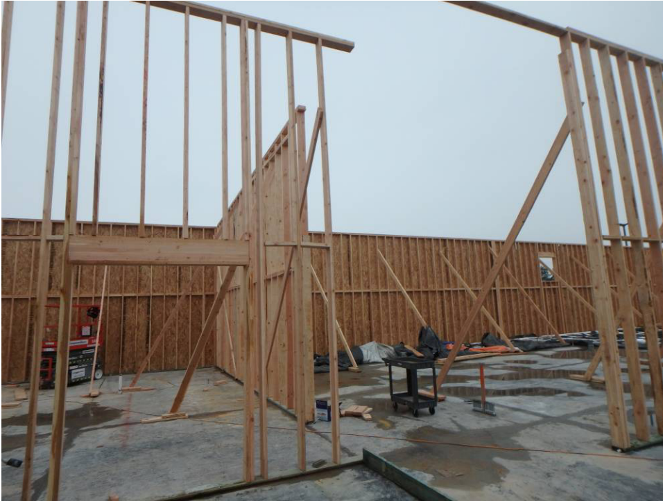
Looking at the west wall framing and sheathing
