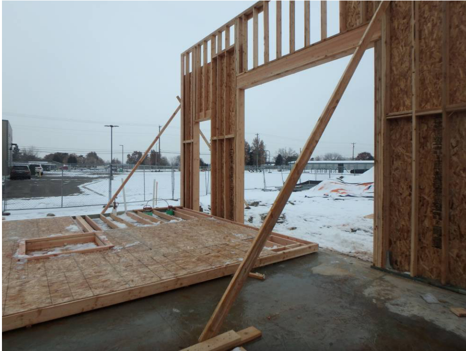
Looking at the northeast corner and the north wall framed and ready to set in place
