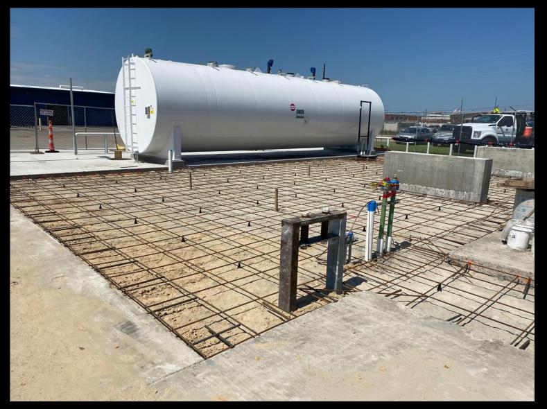
Cre R Installed Diesel-Unleaded fuel tank on concrete base. Rebar for Propane tank is ready for concrete.
