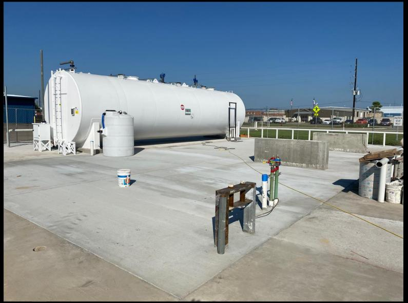
cre R Installed Diesel-Unleaded fuel tank on concrete base. Concrete paving now complete.
