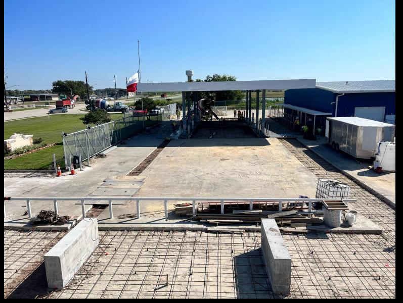
cre R Fueling Station – Canopy Complete– Underground Piping Complete, Paving, Setting Tanks & Equipment to Follow
