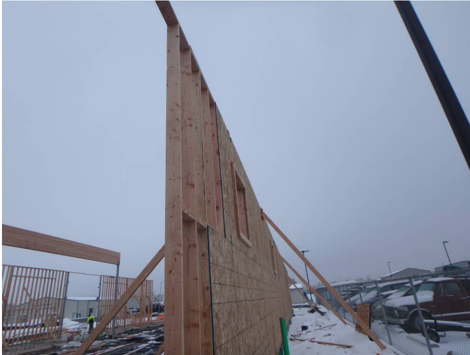
West wall openings and Framing offset
