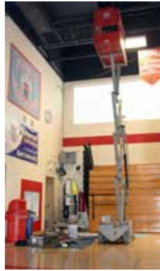
Air Handler NCHS Gym
