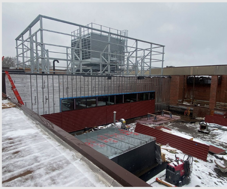
On the multipurpose addition, the enclosure is nearly complete as crews finish installing the metal panels for the final layer of the exterior façade
