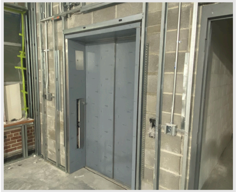
Crews are nearly complete with the installation of the new elevator in the multipurpose addition and lower-level locker room areas
