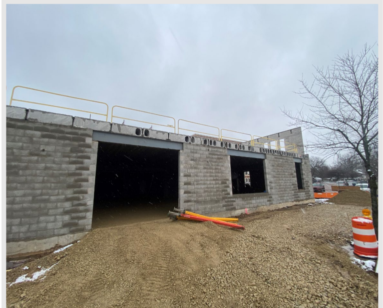
The CMU walls are being constructed on the second level of the cafeteria addition
