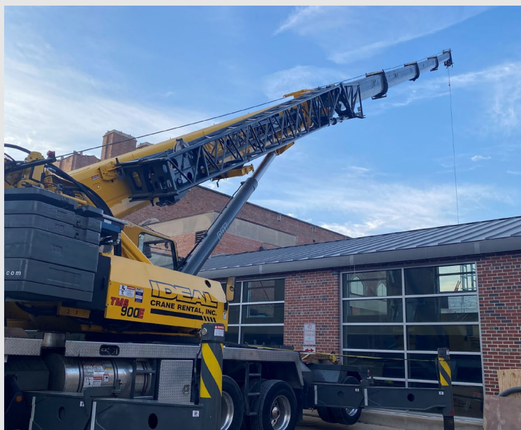
The construction team uses cranes at East High School to safely hoist equipment and materials on-site for the renovation work
