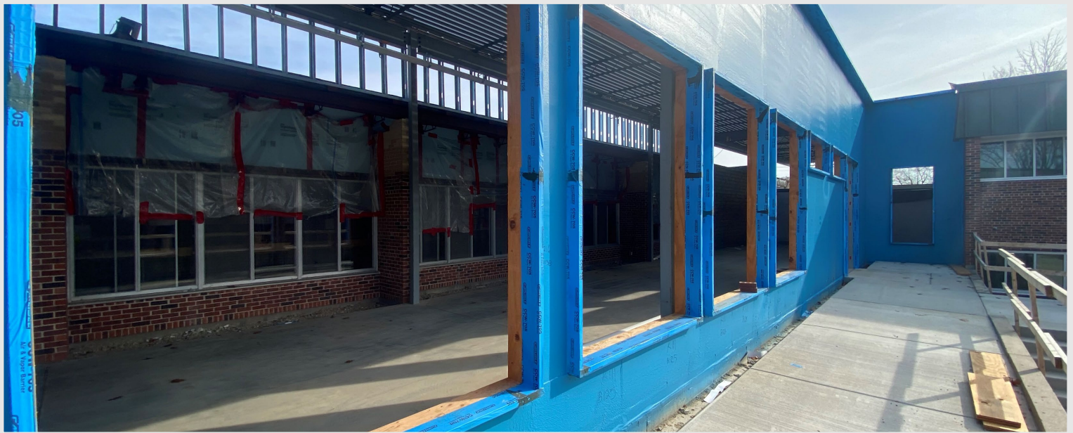
The spray-on exterior vapor barrier has been applied to the new addition
