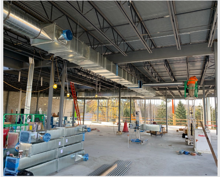
Workers have started installing ductwork throughout the building
