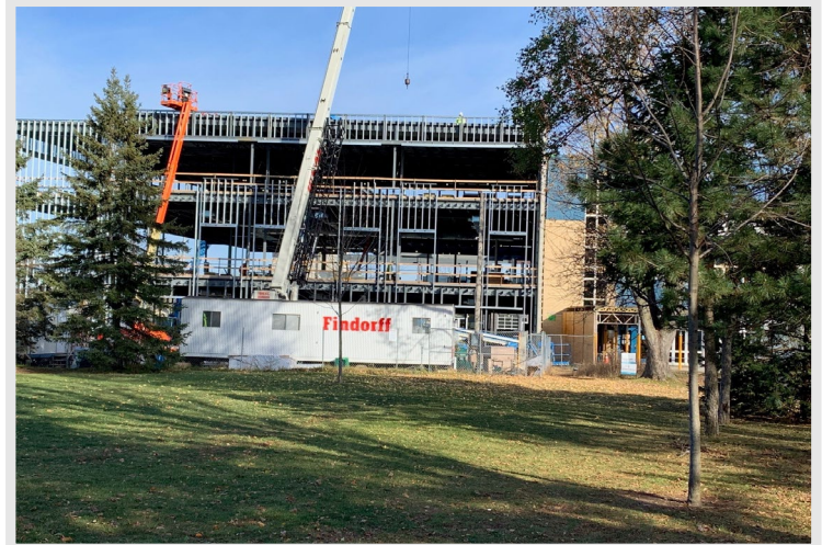
Overall view of the building from the south side
