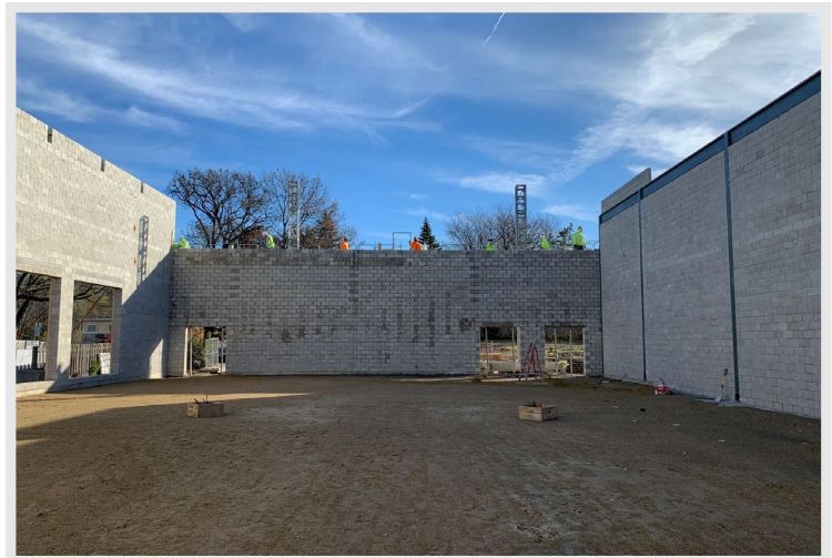
Masons are installing the CMU blocks to construct the last wall of the gym
