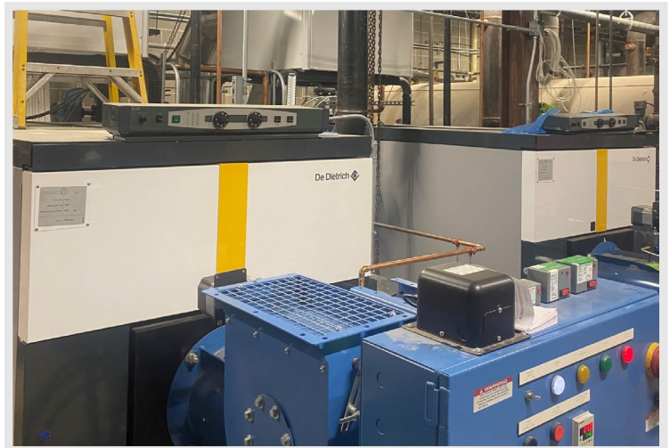
The new boiler system was installed in the mechanical room
