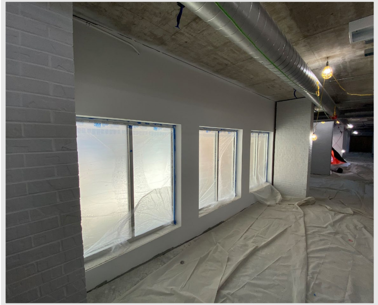
The first coat of paint is being applied in 'The Pit' infill
