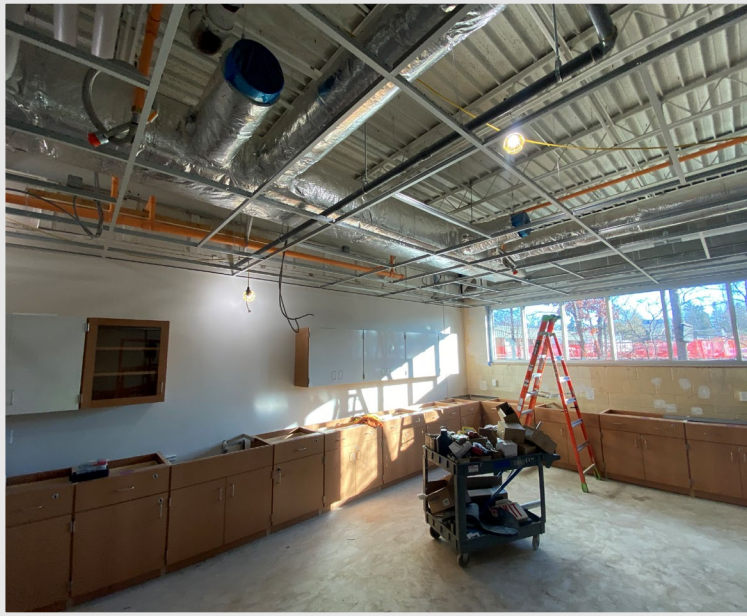
The casework and ceiling grid was installed in the science wing renovation
