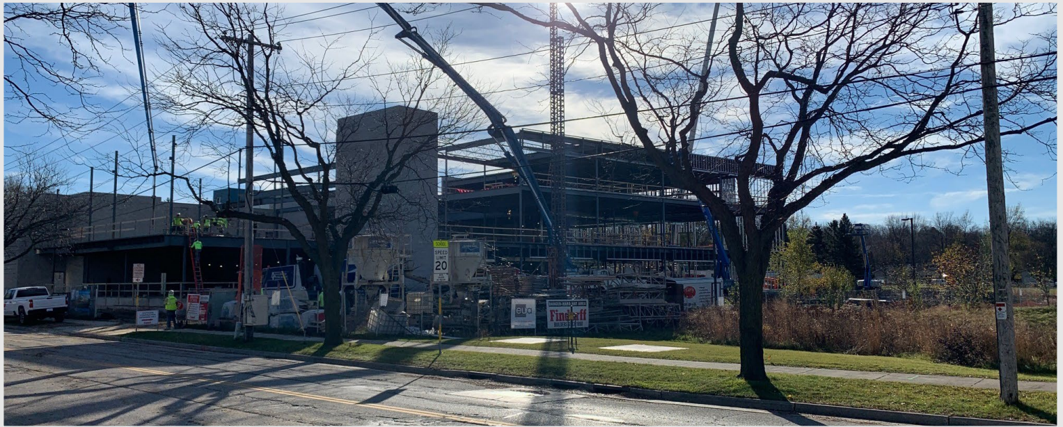
The view of the building progress from the north
