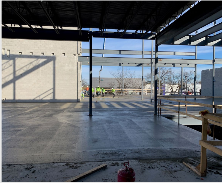
The concrete slab on the north end of the second floor is being poured
