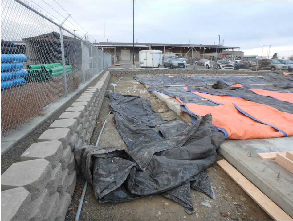
Looking west along the south foundation wall and retaining wall
