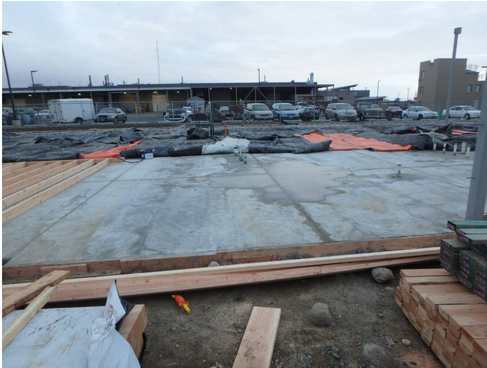
Looking west across the slab and framing
