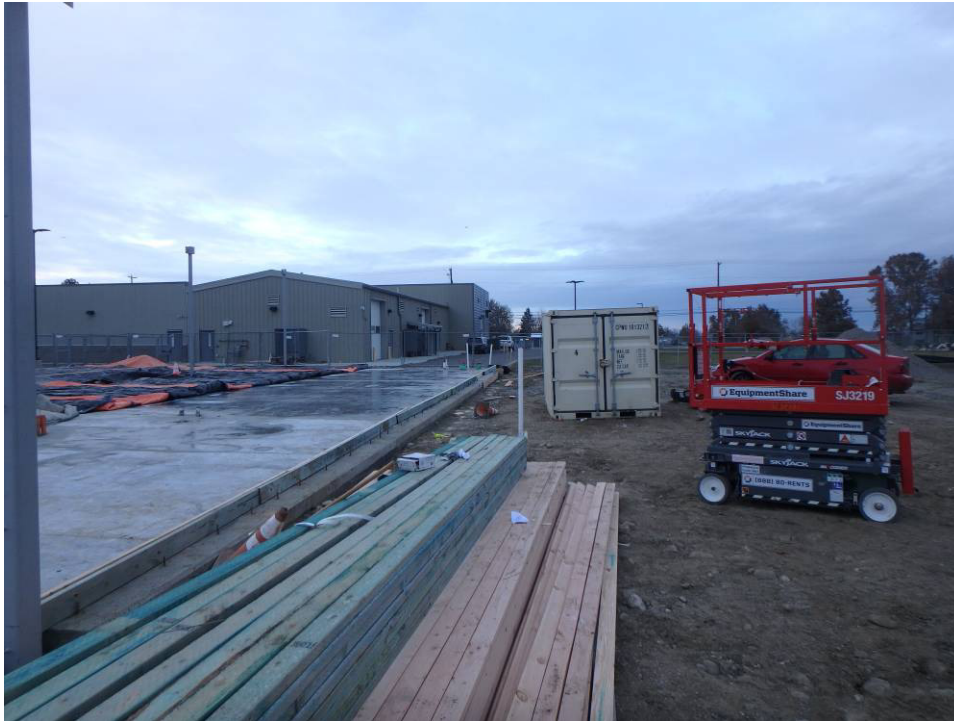
Looking north at the north slab and north east foundation wall
