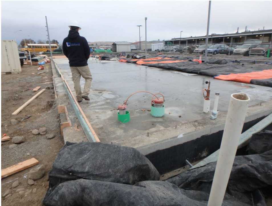
Looking south at the northeast slab building corner
