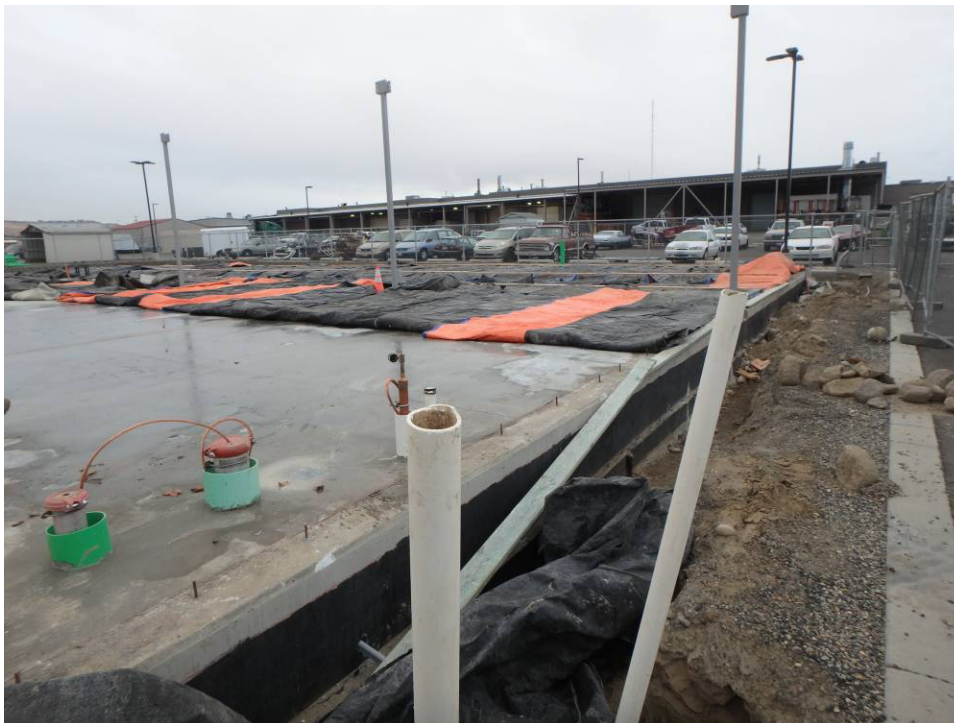
Looking southwest at the north slab and blankets
