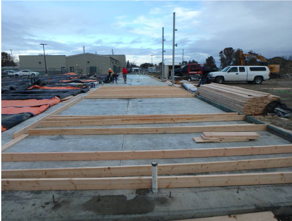
Looking north at the east wall framing from the SE corner
