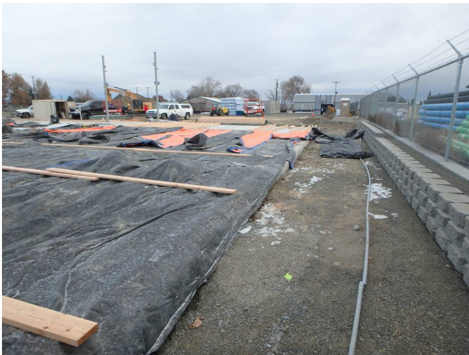
Looking east along the south foundation wall and retaining wall
