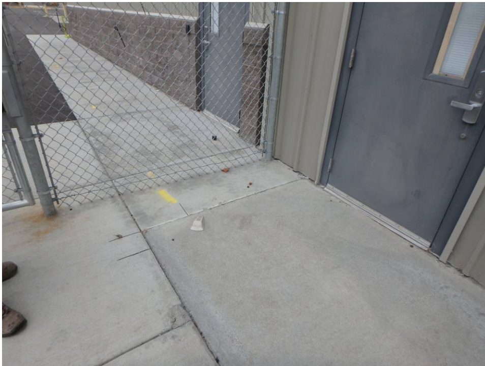
Tri Tech East – slab to be removed, locate and old sawcuts
