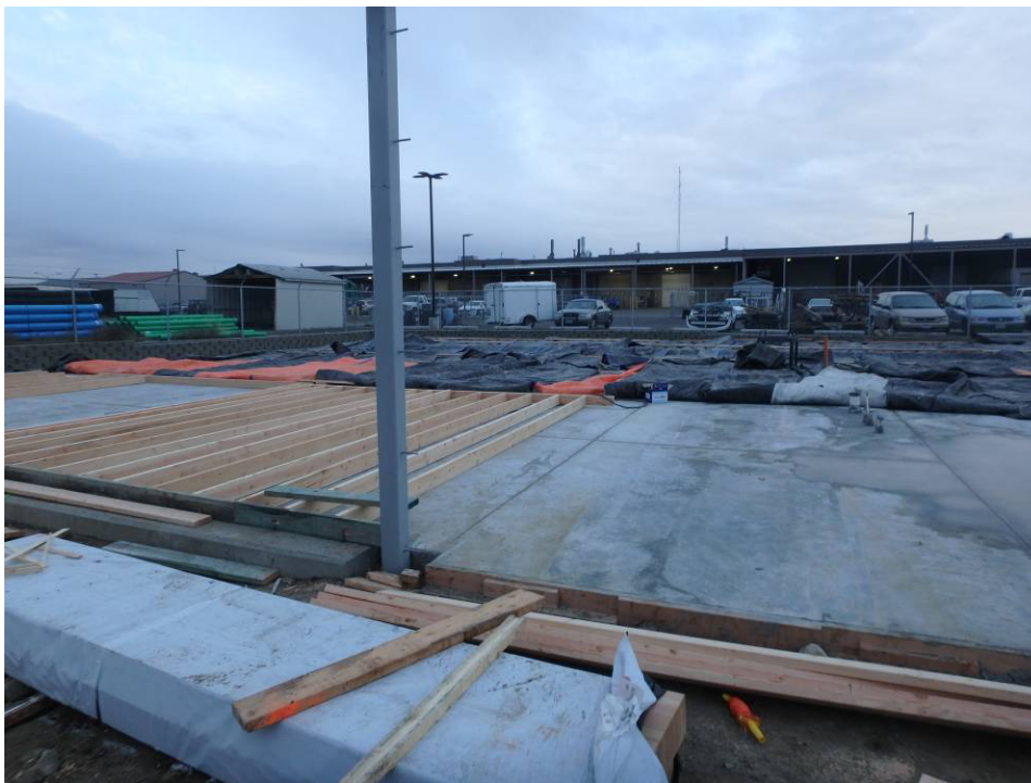
Looking southwest across the slab and framing
