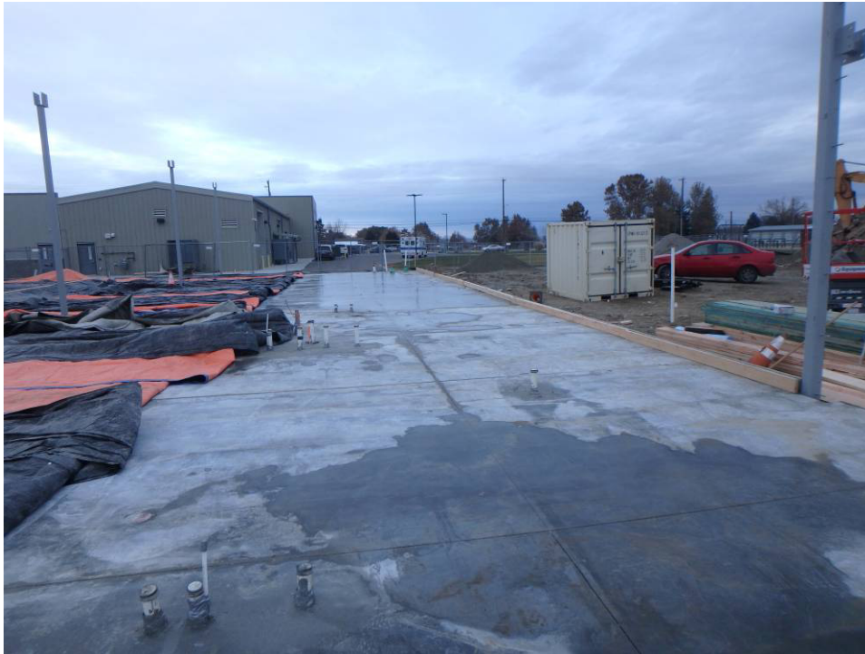
Looking north at the north slab, east side
