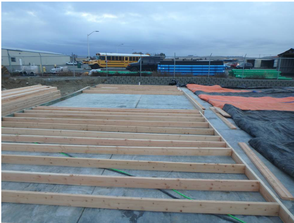
Southeast wall framing
