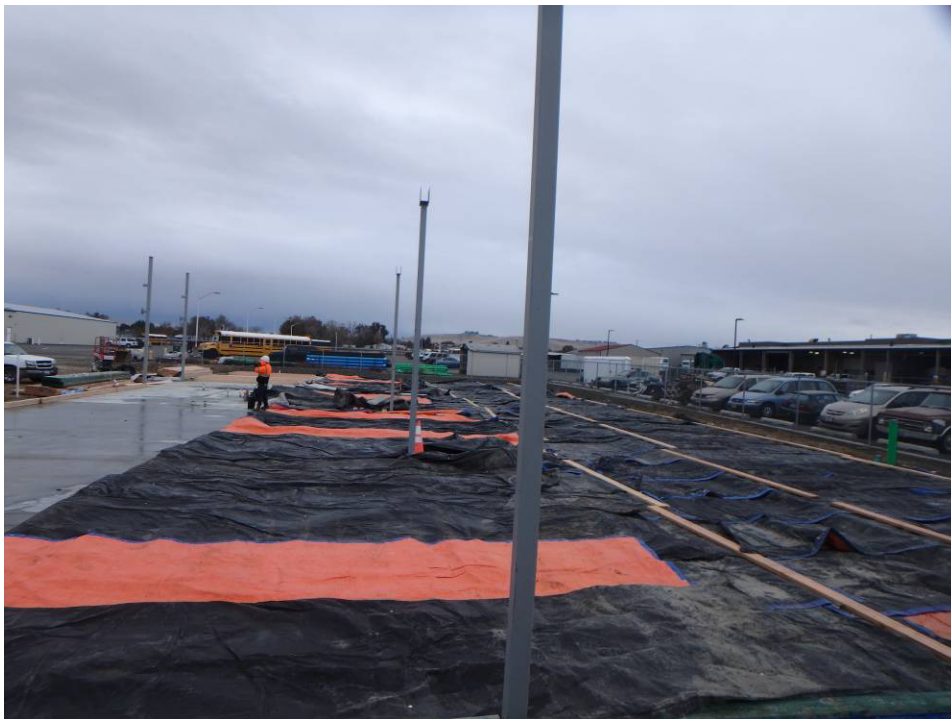
Looking south at the central building area and 3 new north columns
