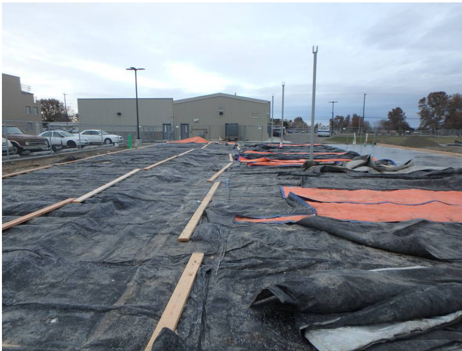
Looking north at the north slab, west side
