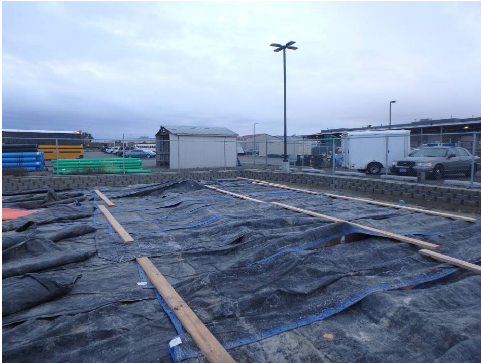
Looking south at the south slab, west side
