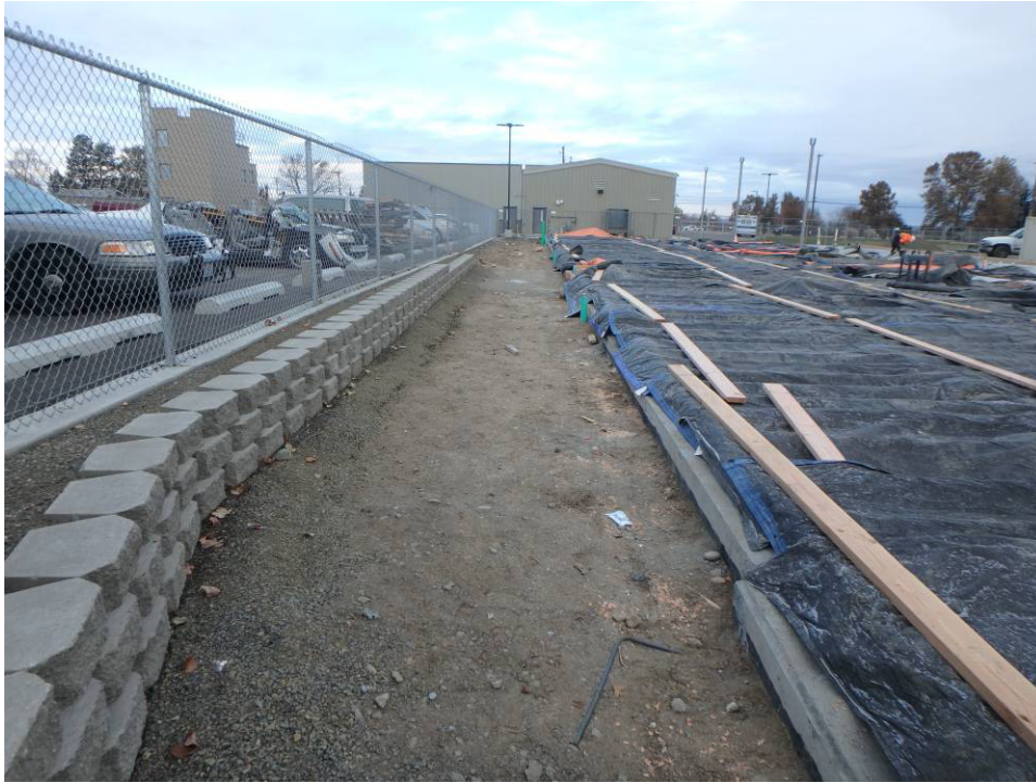
Looking north at the west retaining wall and building slab
