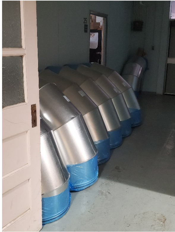
Material Delivery and Staging
