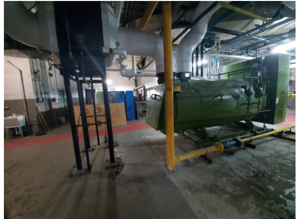
Boiler Room Prior to Work
