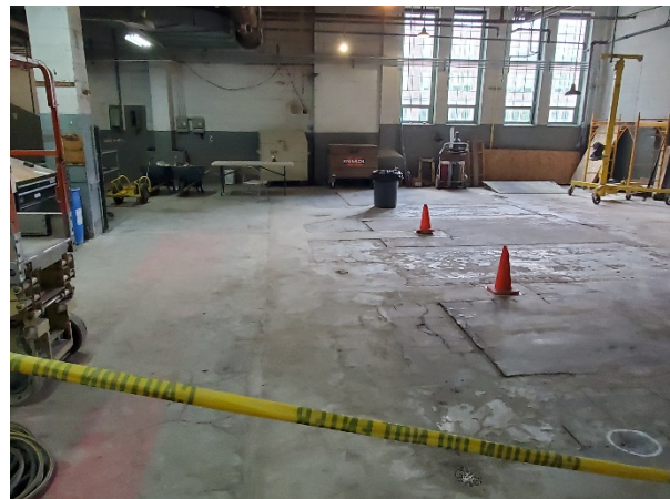
Boiler Room after Demolition
