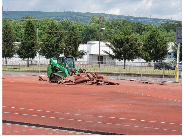
Track Surface Removal
