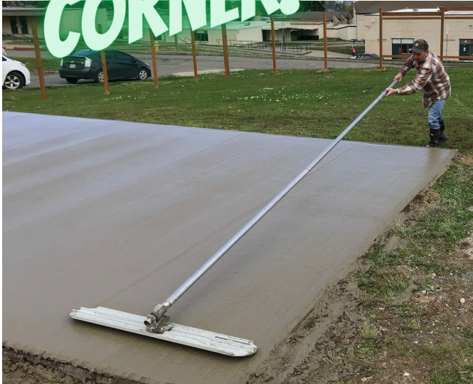
Tim floating concrete for the PAHS Greenhouse
