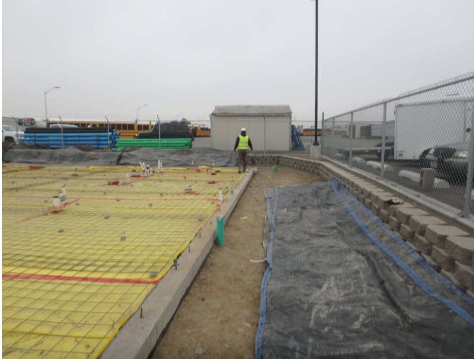
Southwest corner foundation and retaining walls and blanket
