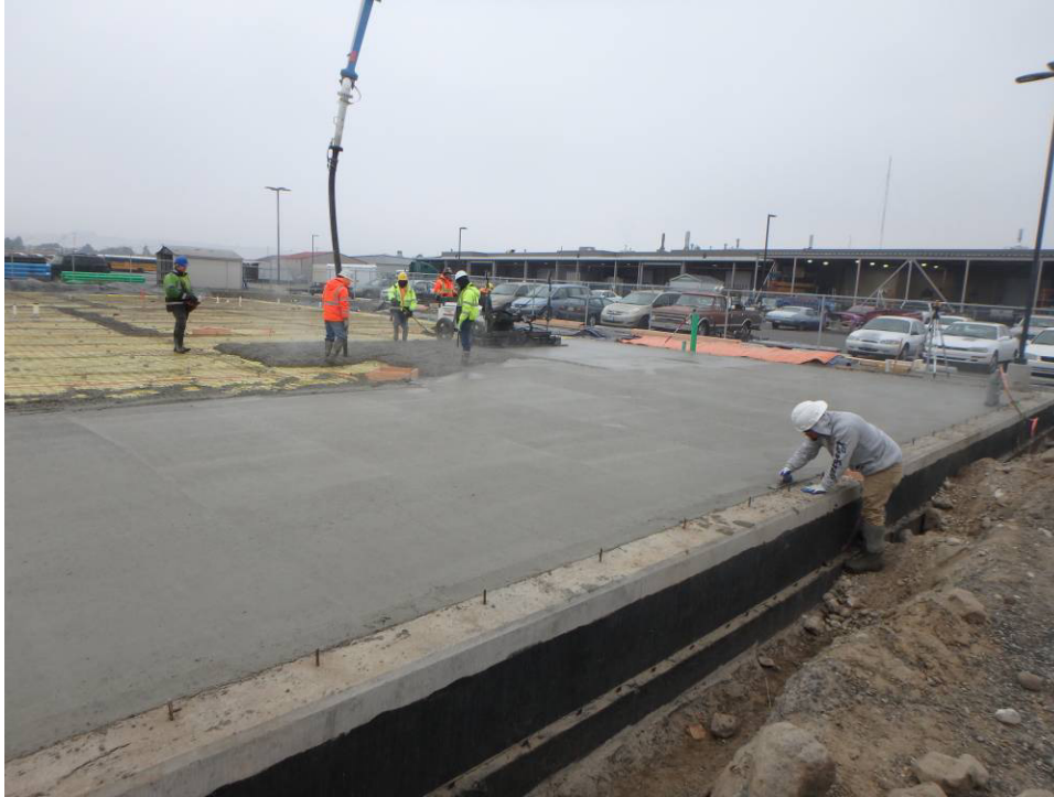
Northwest corner finishing
