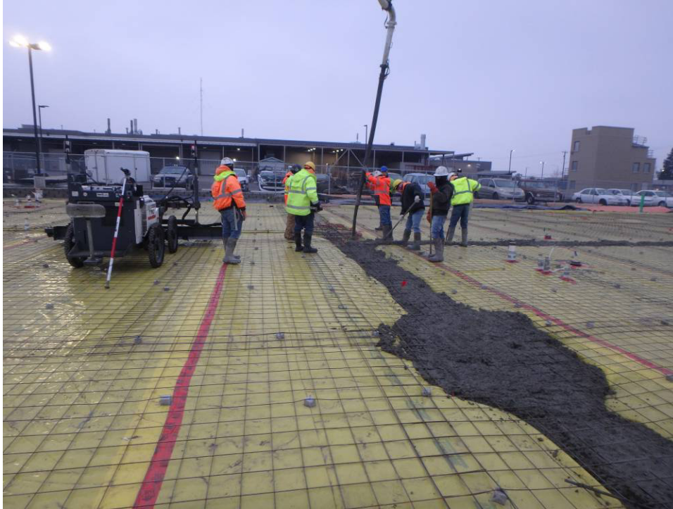
Placing concrete in the central east-west thickened slab area
