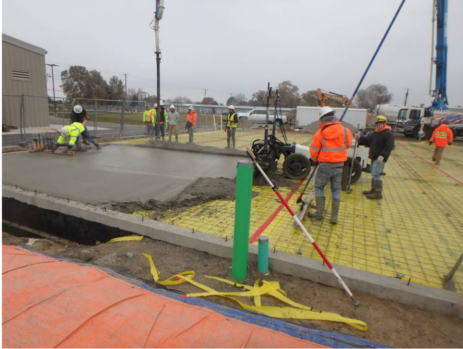
Placing concrete in the northwest corner
