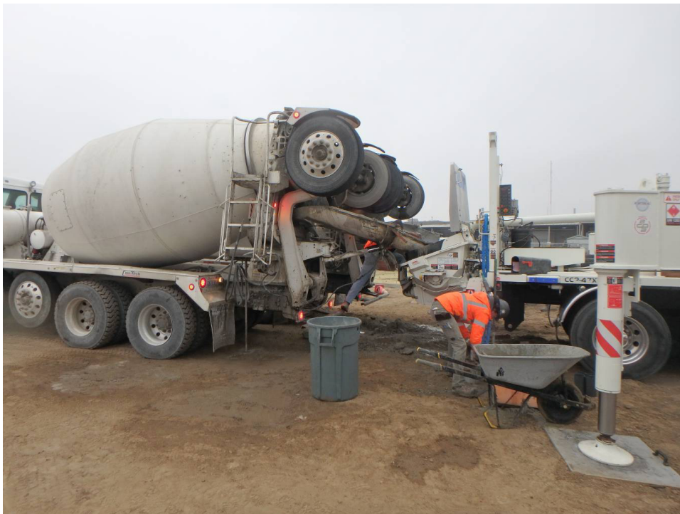
Concrete trucks and taking samples.
