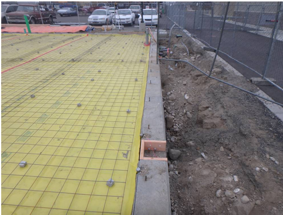
Looking west along the north foundation wall to the northwest corner
