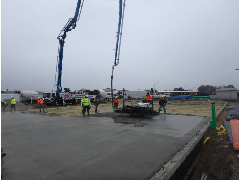
Power screed at north “diamond”
