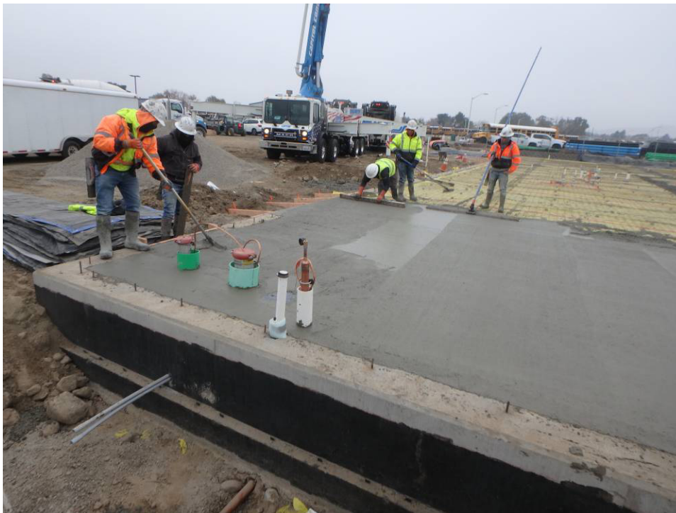
Northeast corner finishing
