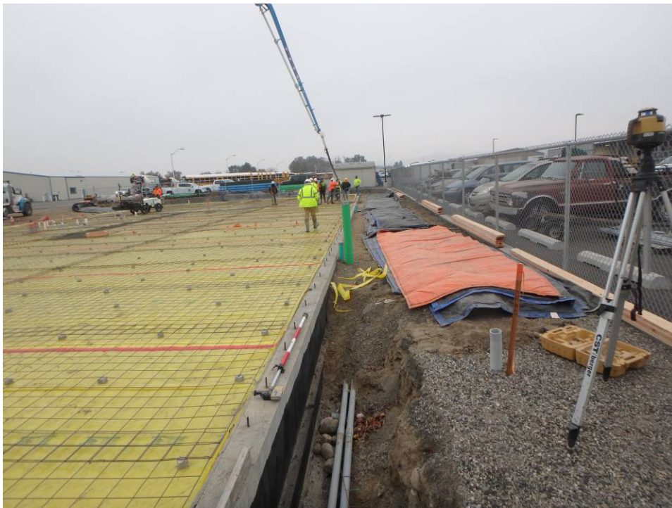
Looking south at the west retaining wall and the crew finishing the thickened slabs
