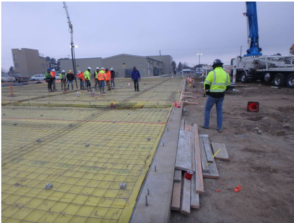
Looking north at the north slab area and vapor barrier along the east foundation wall
