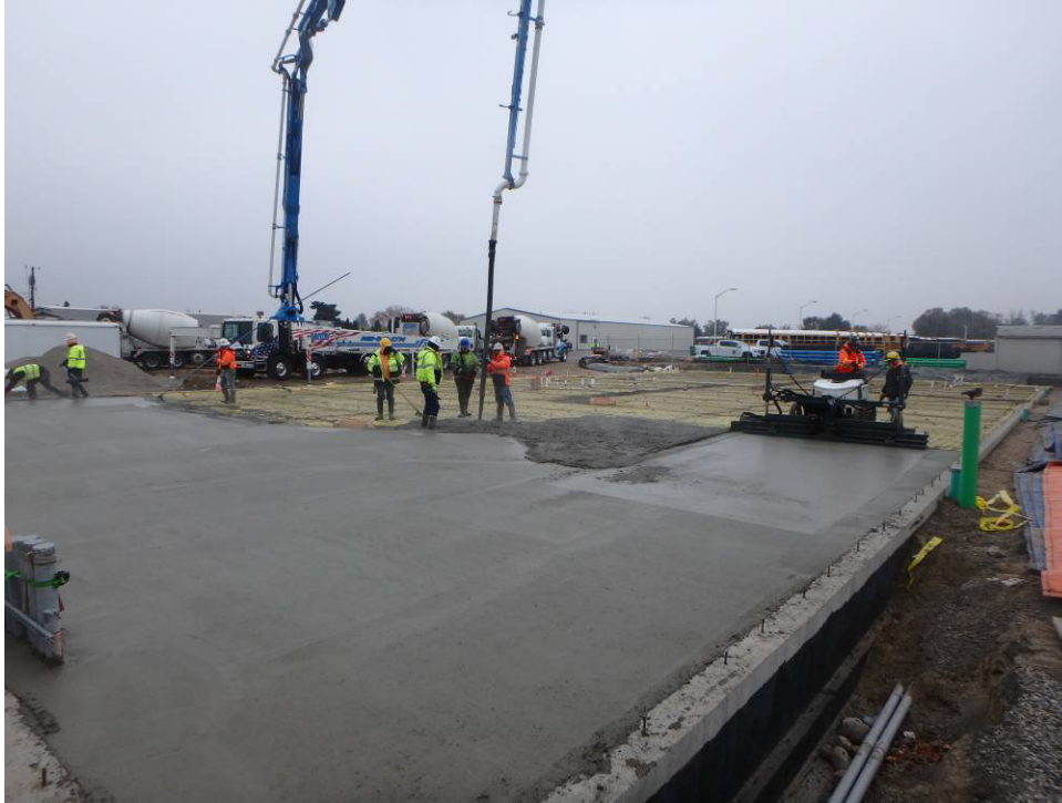
Placing concrete
