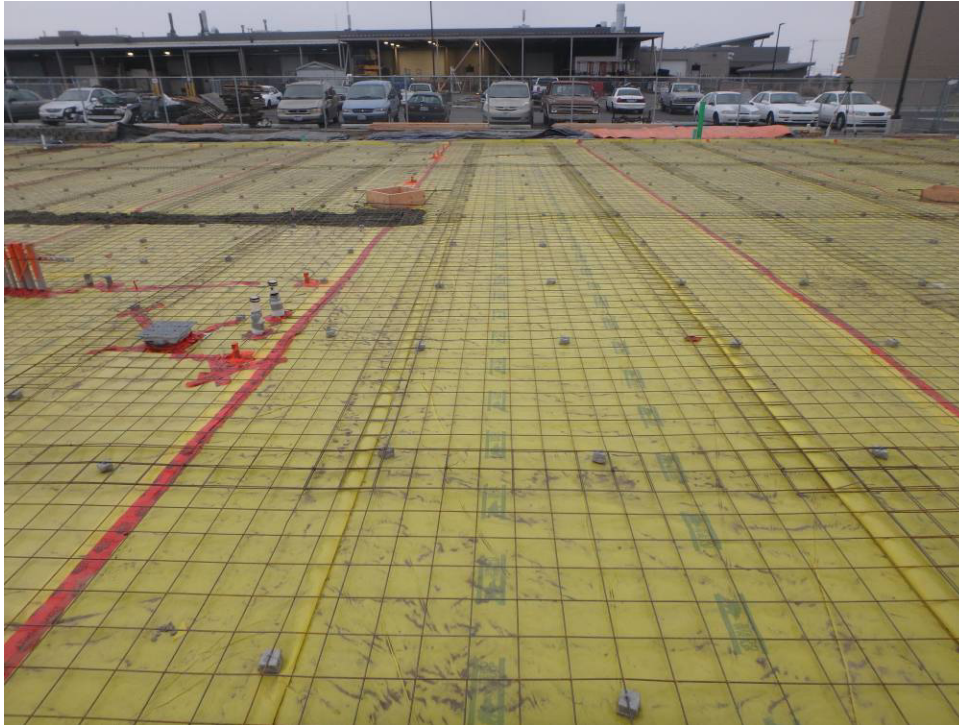
Vapor barrier sheeting, welded wire fabric and chairs
