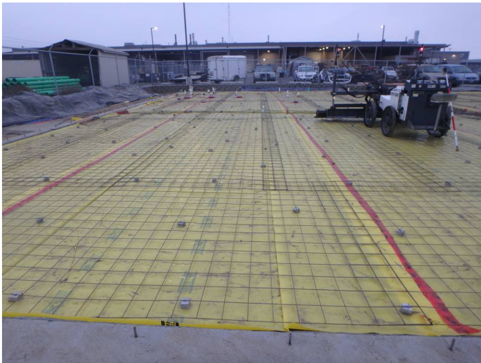
Looking west along the south foundation wall
