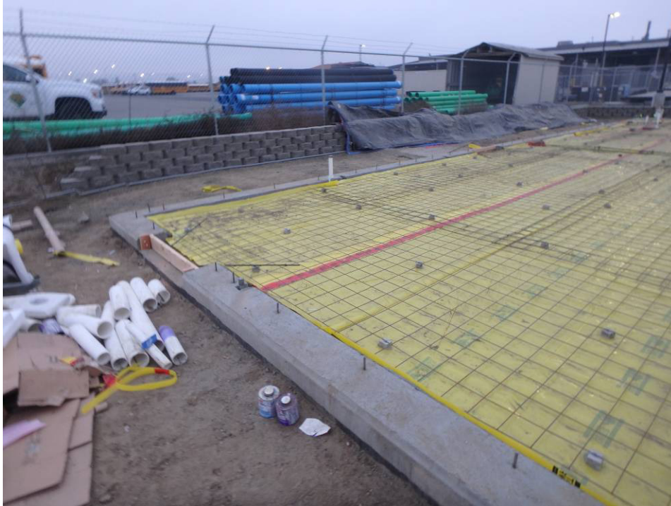
Southeast corner of the slab with vapor barrier, weld wire mesh and hairpin rebar
