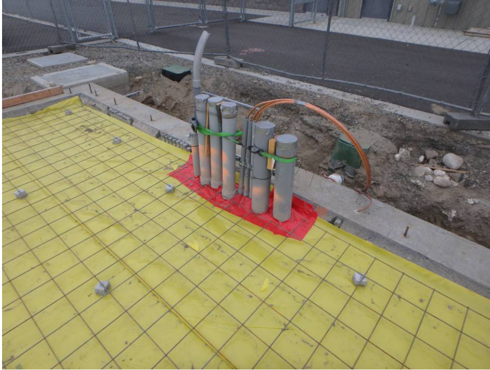
Conduit stub up in the northwest corner
