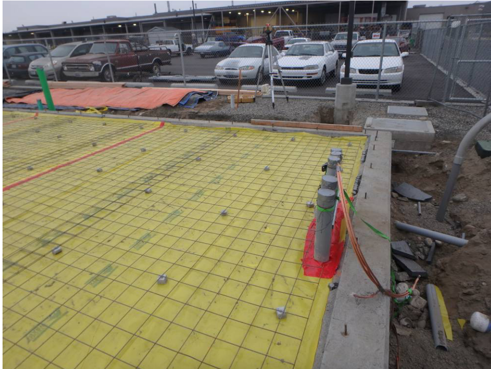
Looking west at the northwest corner of the foundation wall and the vapor barrier and welded wire mesh
