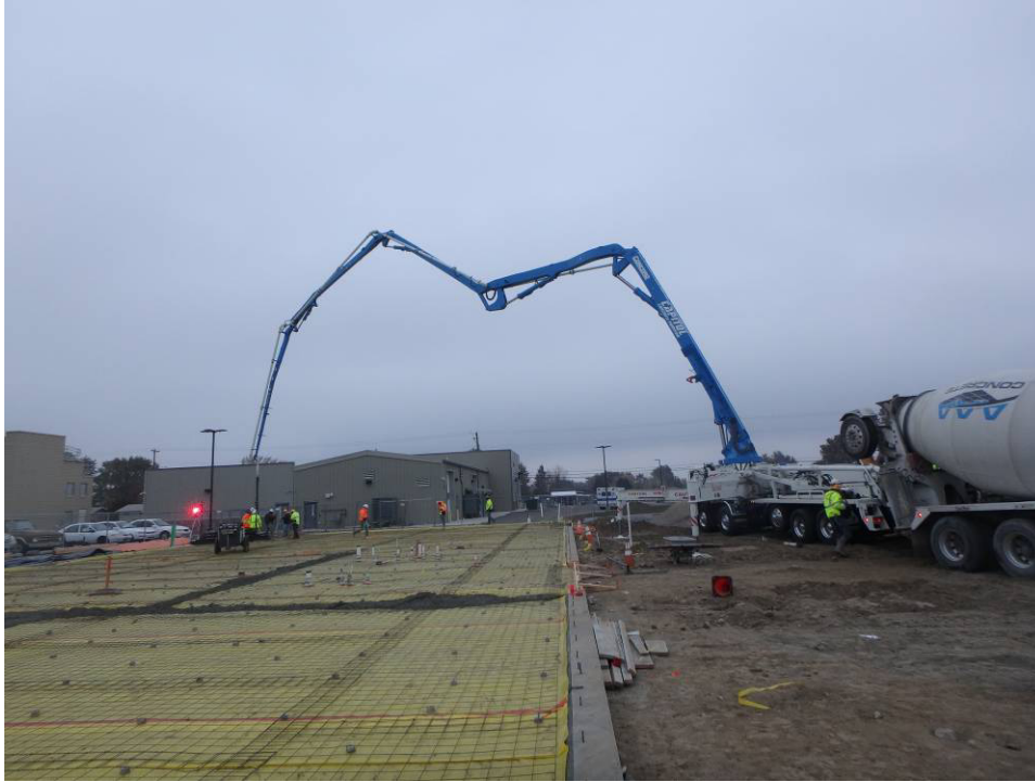
Moving to placing concrete in the northwest corner of the building
