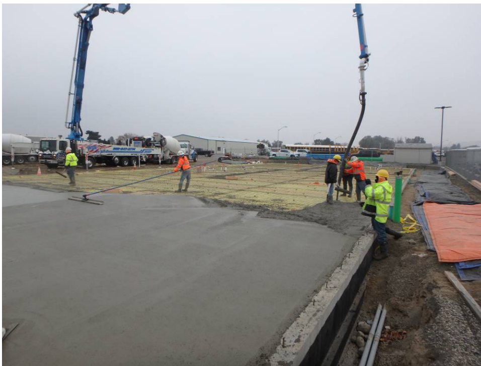
Moving south placing concrete
