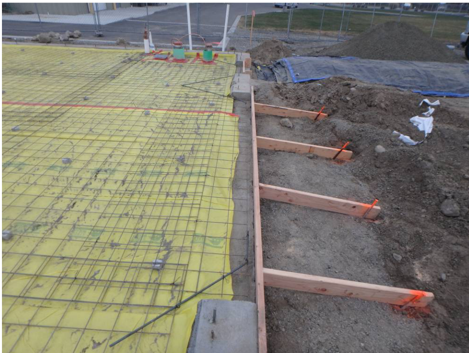
Looking northeast corner at the north end vapor barrier
