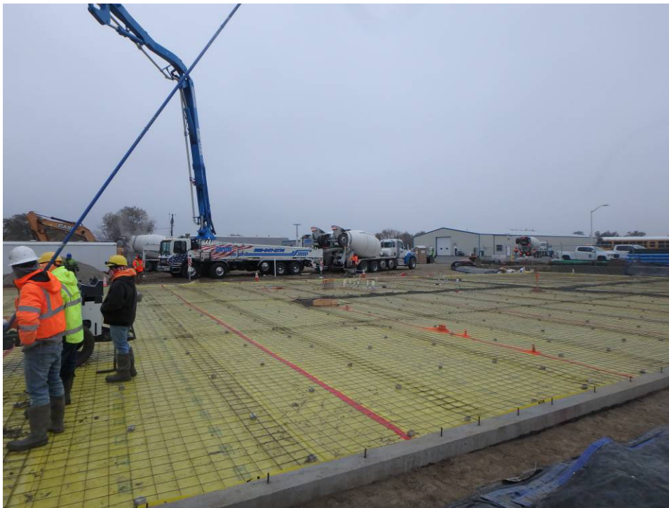
Looking southeast across the building footprint, ready for concrete
