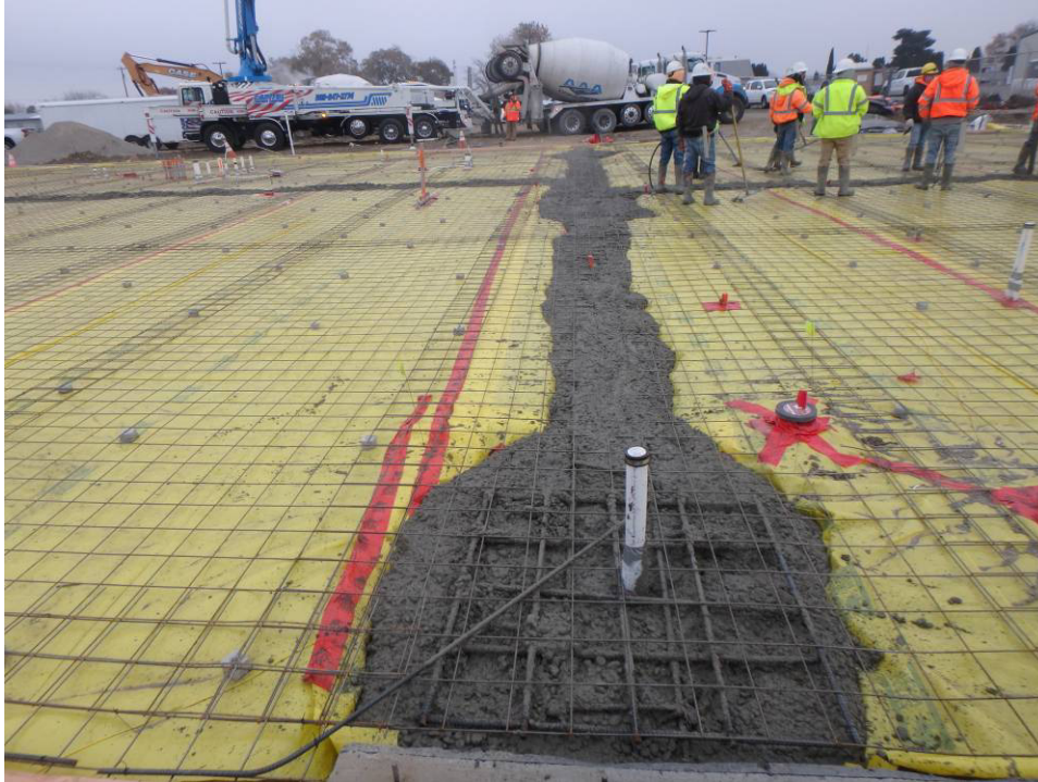
Thickened slab trench concrete in place
