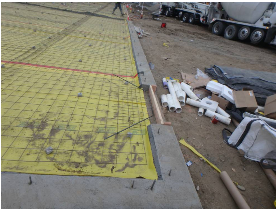
Looking north at southeast corner and the east foundation wall
