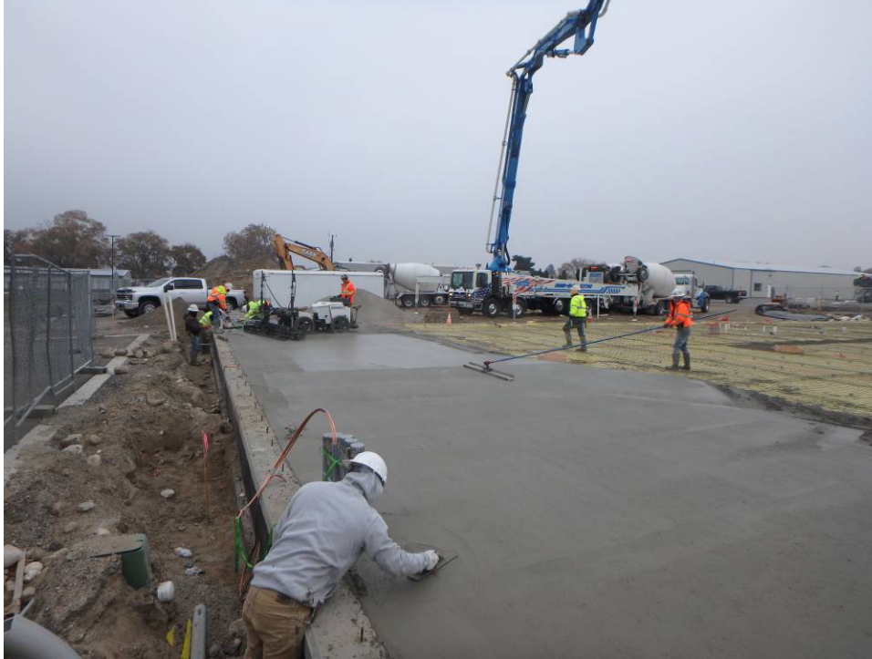
Concrete placed across the north edge of the building
