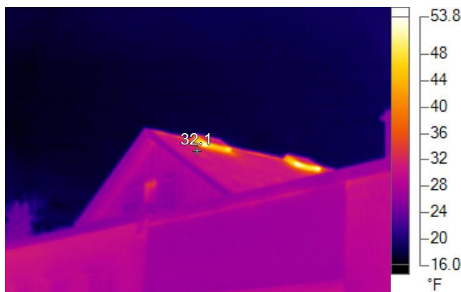
Figure 6: Infrared Image of heat loss through the skylights in the art studio.
