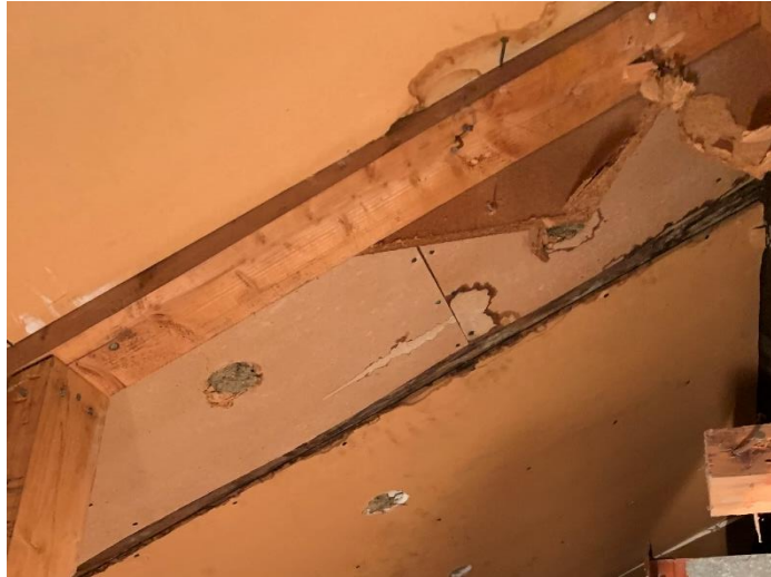
Figure 2: Water damage on the existing paper board in the attic.
