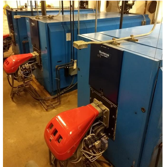
The existing oil-fired boilers
