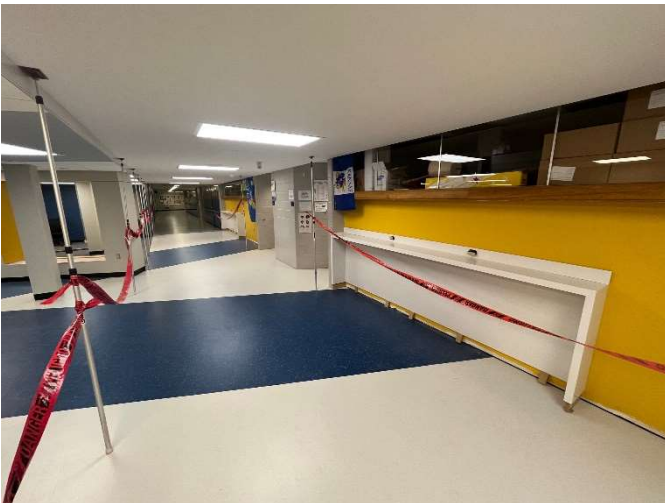
Solid surface installation in Level 1
