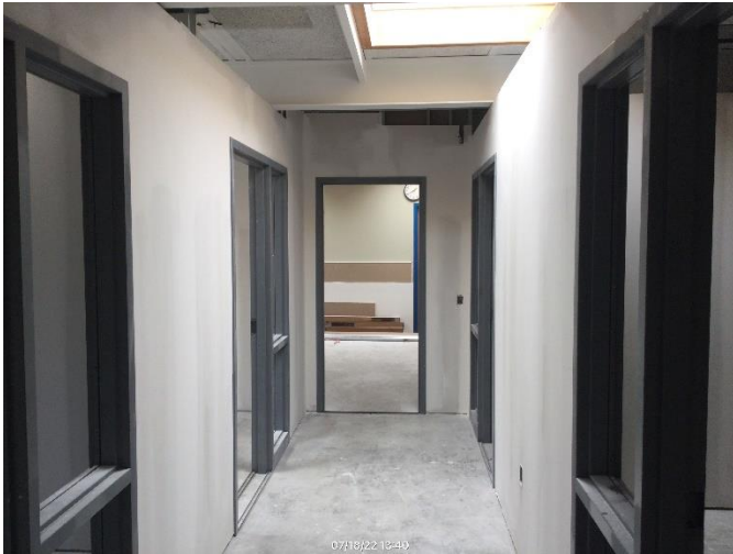
Finishing drywall and doorframe installation in 2 nd floor offices
