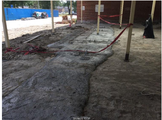
Poured footing in 2 nd floor addition
