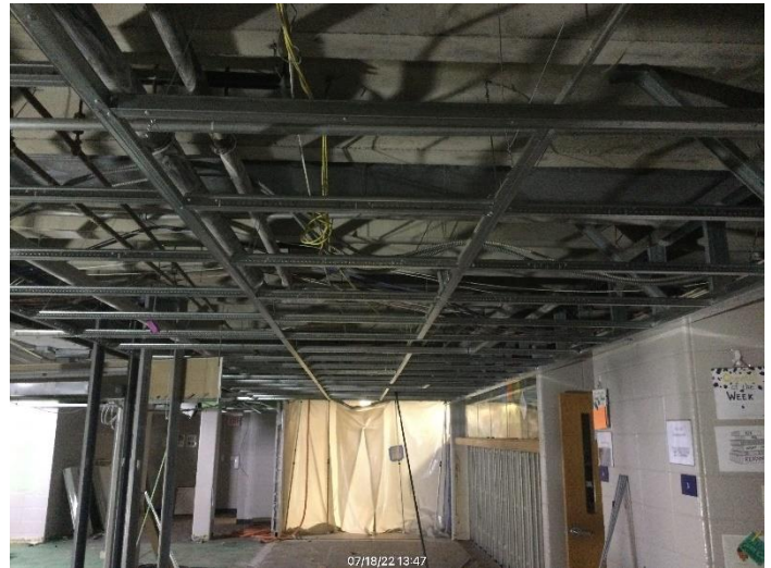
Installation of corridor ceiling grid in 1 st floor area
