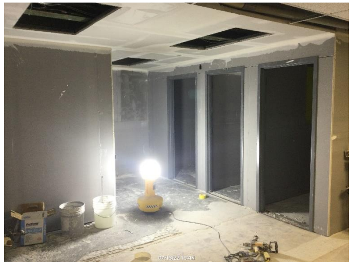
Continuing drywall installation in 2 nd floor bathrooms
