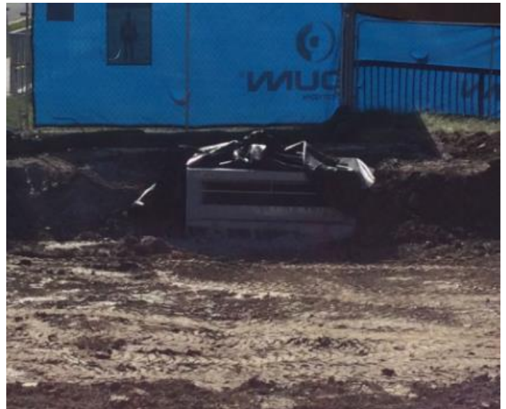
Storm Inlet SW Corner
