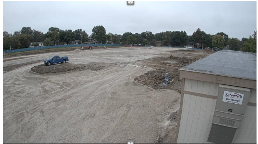
Overview of Jobsite
