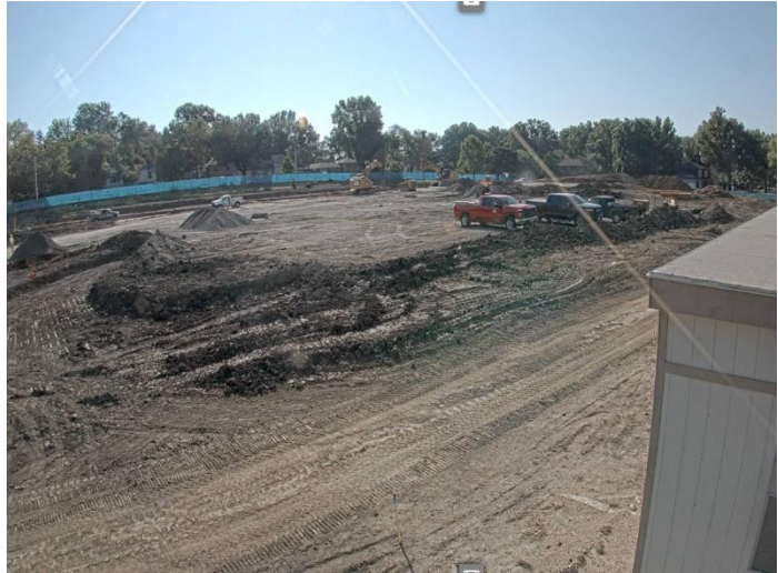
Overview of Jobsite
