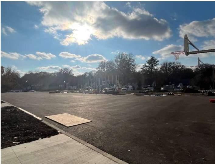
Begin playground equipment install
