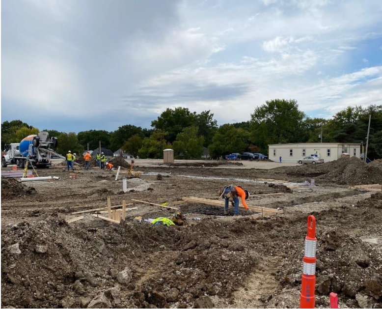
Area D Footing Preparation
