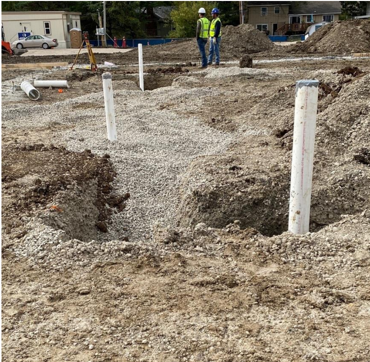
Area D Storm Line
