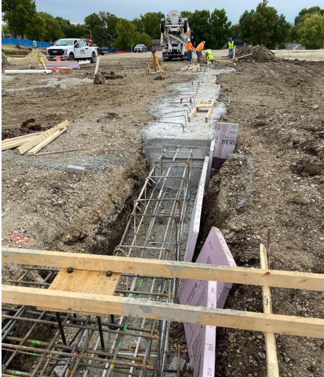
North End Area D Footings
