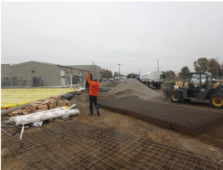
Moving the welded wire mesh reinforcement into place
