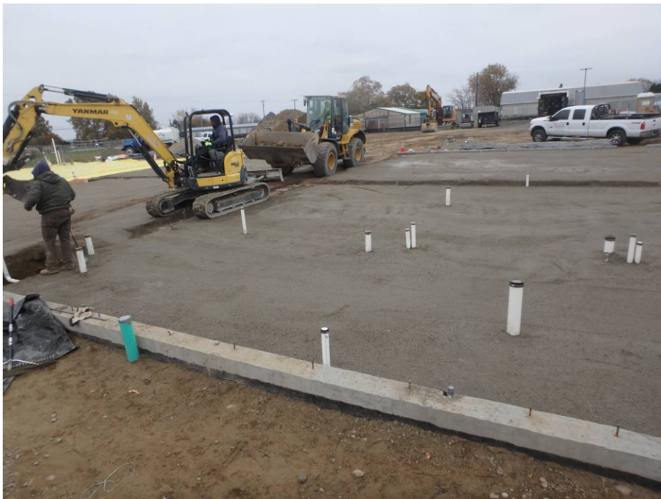
Thickened slab trench digging
