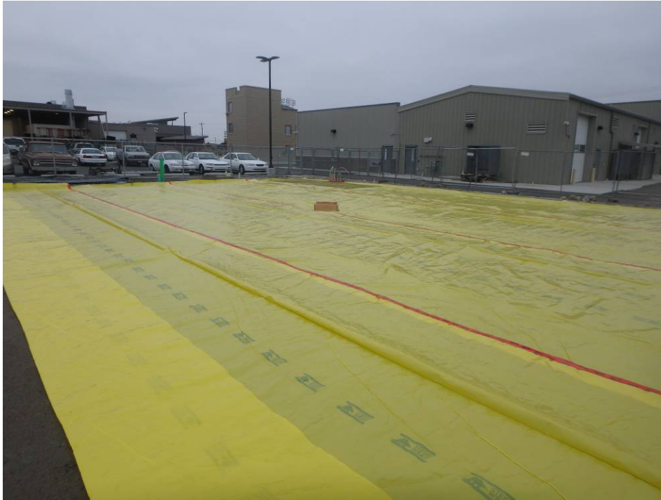
Looking northwest at the north end vapor barrier
