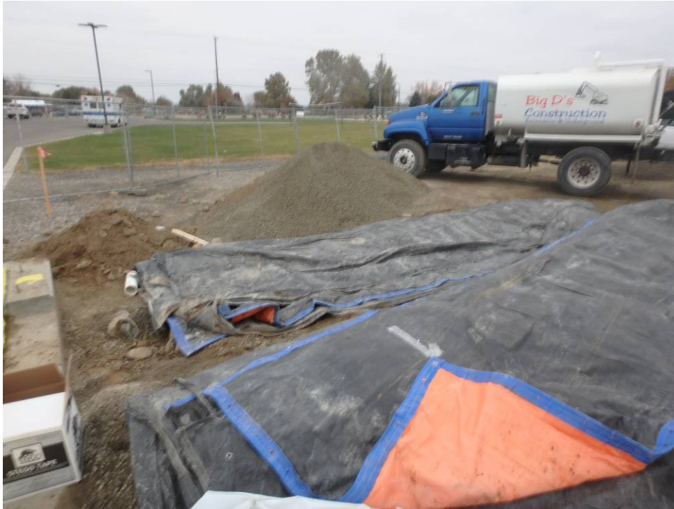
Slab/ soil warming blankets
