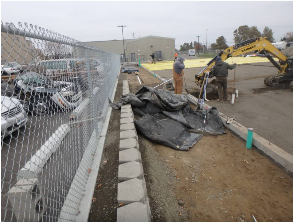
Looking south along the west foundation wall and retaining wall and thickened slab trench digging
