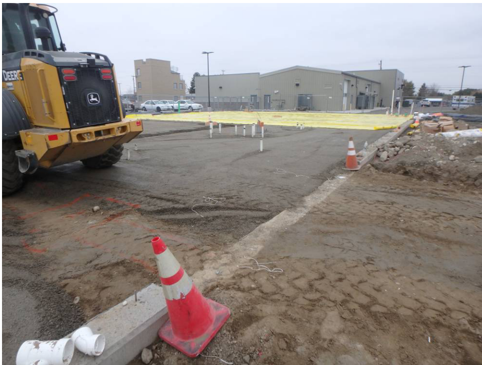
Looking north at the north slab area and vapor barrier
