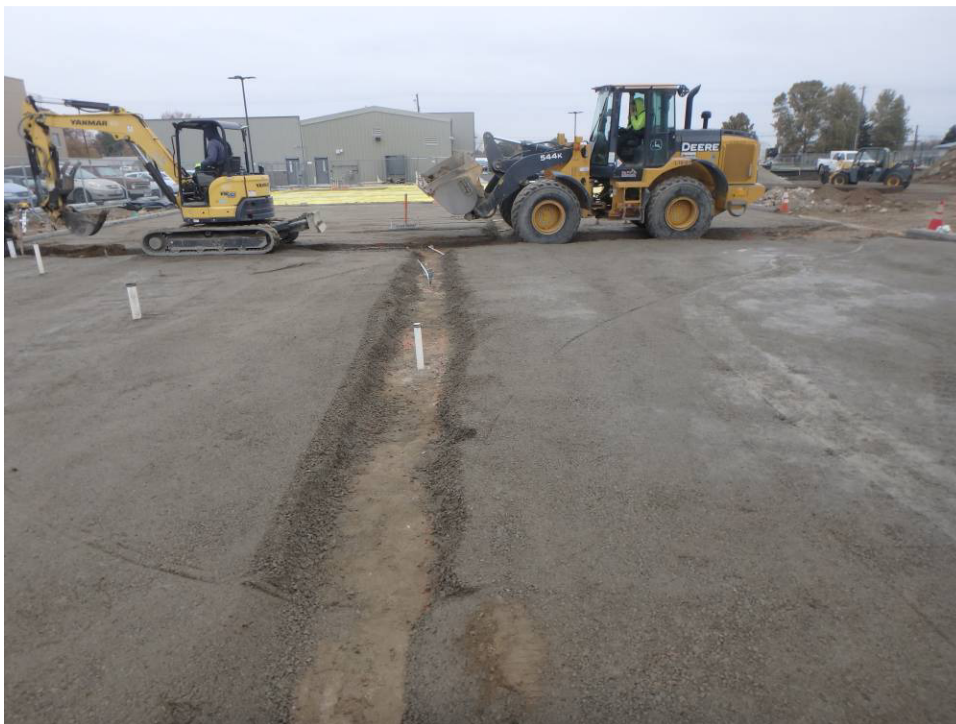
Looking north across the building footprint and the central thickened edge trench
