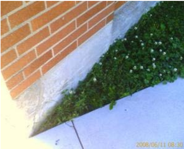
Typical Cast-in-Place Concrete Foundation Wall
