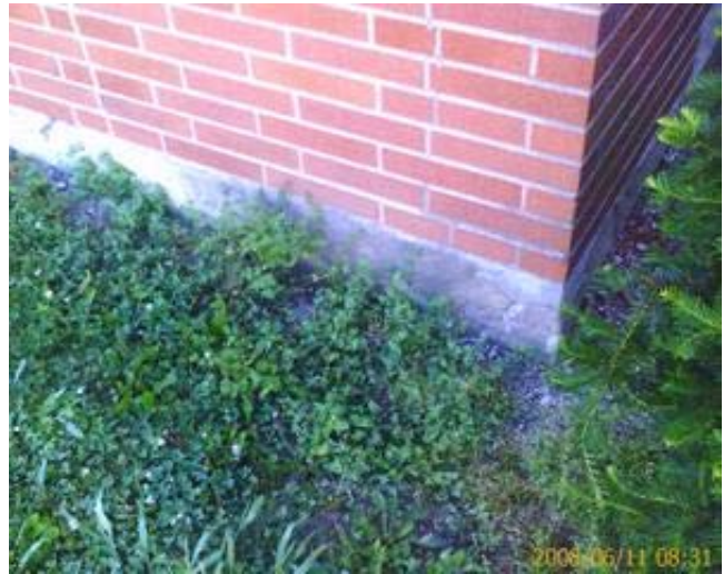
Typical Concrete Masonry Unit Foundation Wall
