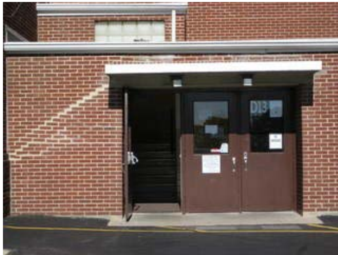
Typical Exterior Doors
