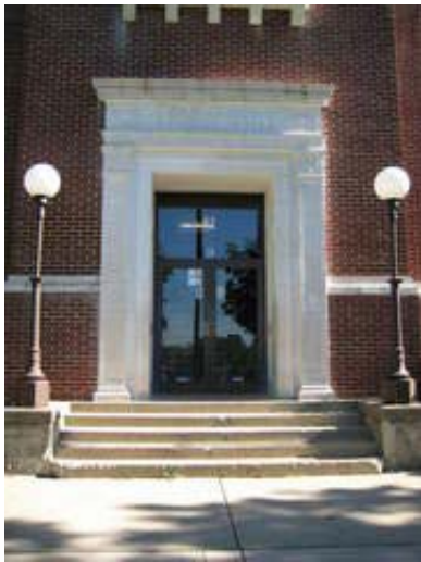
Main Entrance Doors
