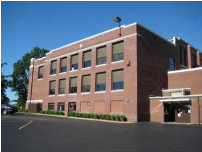
Typical Aluminum Frame Windows
