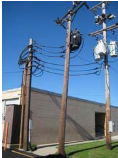
Pole-Mounted Transformers
