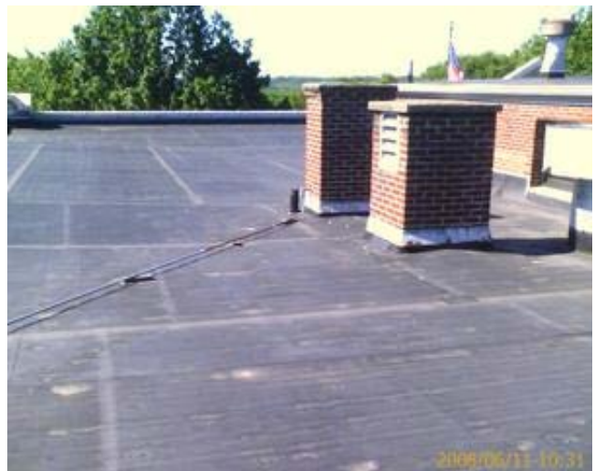
Typical EPDM Roofing Condition
