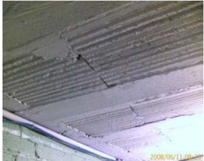
Typical Cast-in-Place Concrete Intermediate Floor
