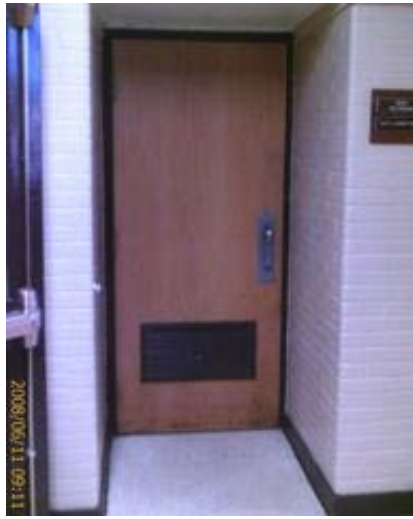
Typical Narrow Recessed Door
