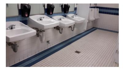
**WATER CLOSETS/URINALS:** The majority of the water closets in the school have automatic sensor flushometer valves. This is also true for the urinals. There is one ganged toilet room that has four waterless urinals (see below). The Boy's Room (2<sup>nd</sup> floor of the original building) was renovated during the 2002 renovations but no privacy screen was installed between the urinals (see below).
