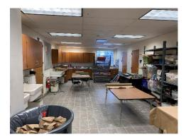
The transition between the VCT flooring in the "instructional" section of the room and the quarry tile on the floor in the rear of room (where the sinks are located) is quite noticeable due to a difference in the elevations of the floors. The quarry tile extremely difficult to clean.
