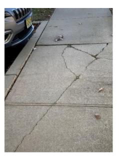
The concrete in the ramp up to main entrance has noticeable cracks running from side to side and should be monitored.
