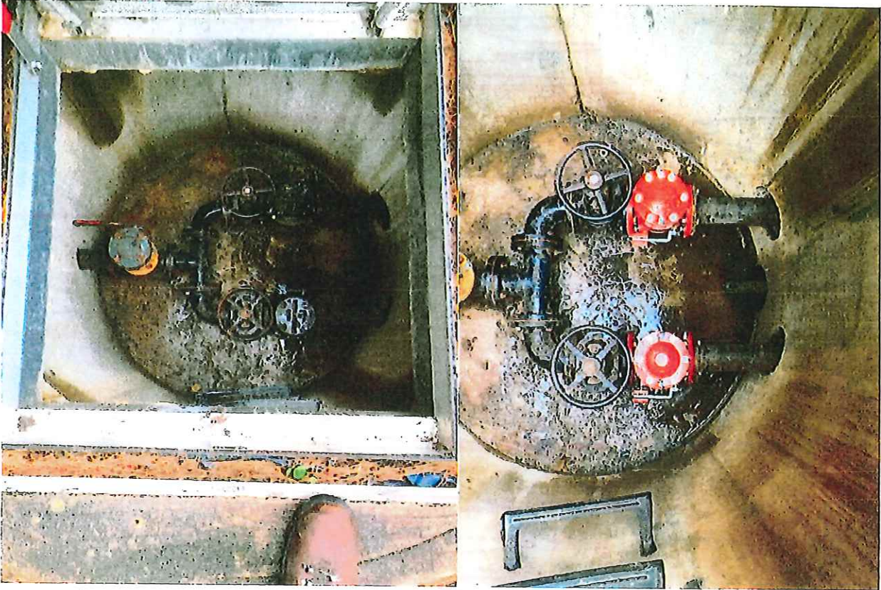
WPCA Operators Installed New Check Valves at PS #16 (Prospect Street)
