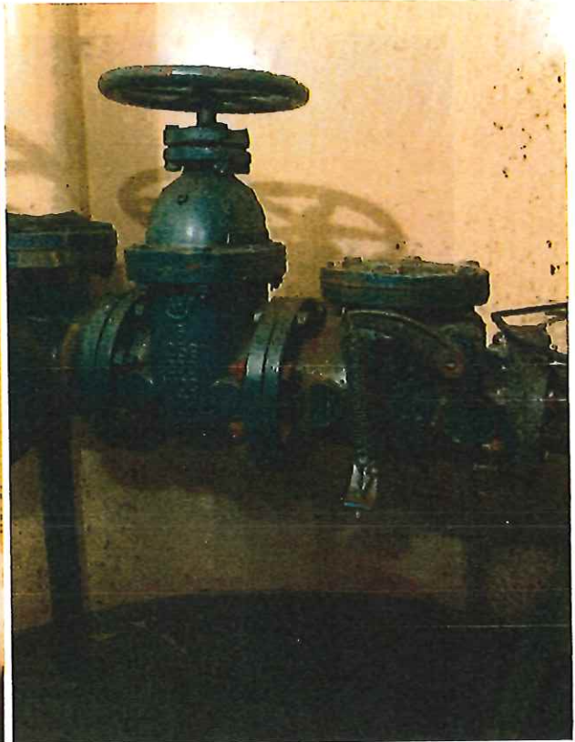
New Suction, Discharge, and Check Valves were installed for both Pumps at PS #6
