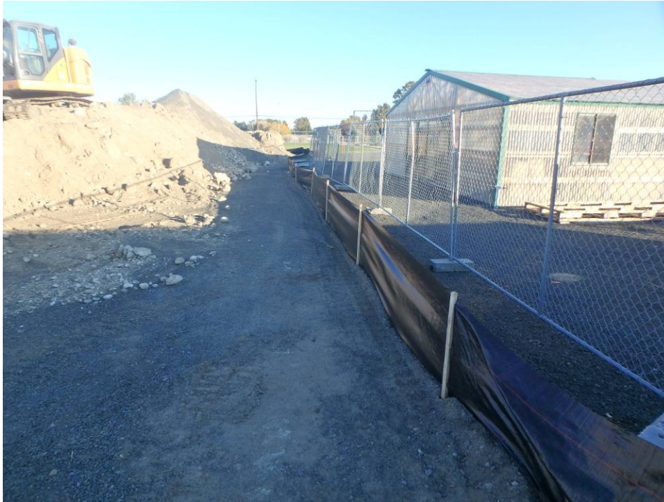
Looking north at the Silt fence towards the northeast corner of the site
