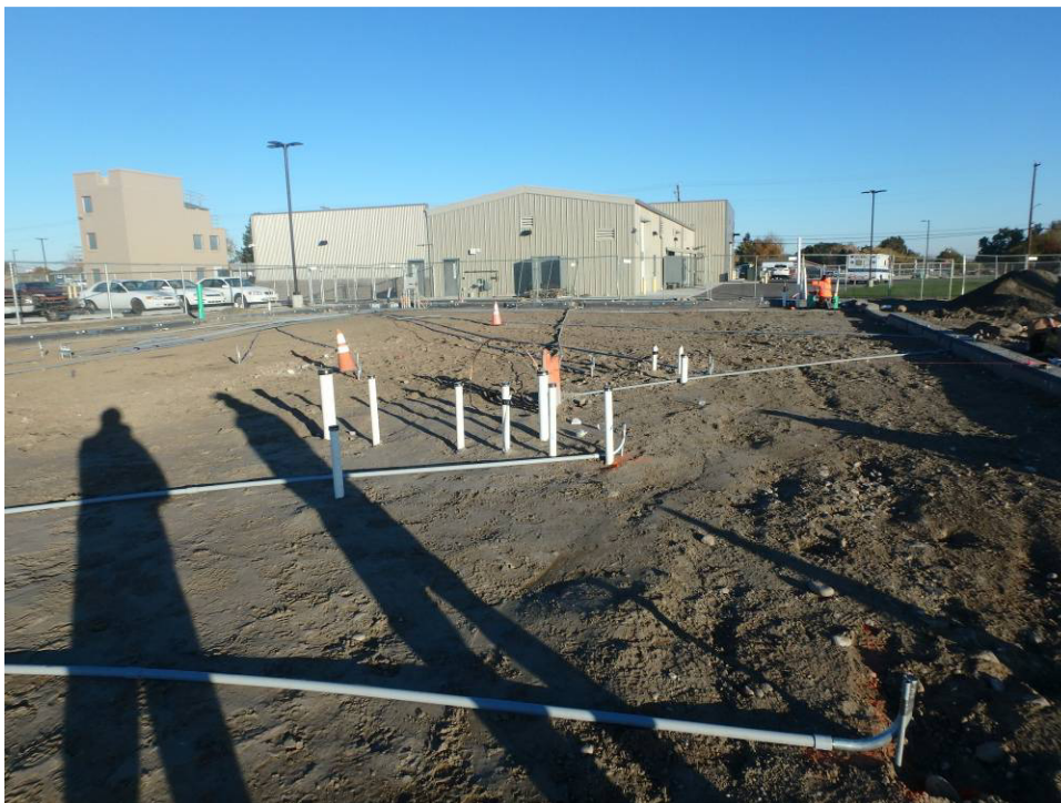
Looking north at the north half of the building and stub-ups
