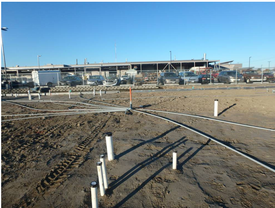
Looking west at the north sub-slab conduit from the center
