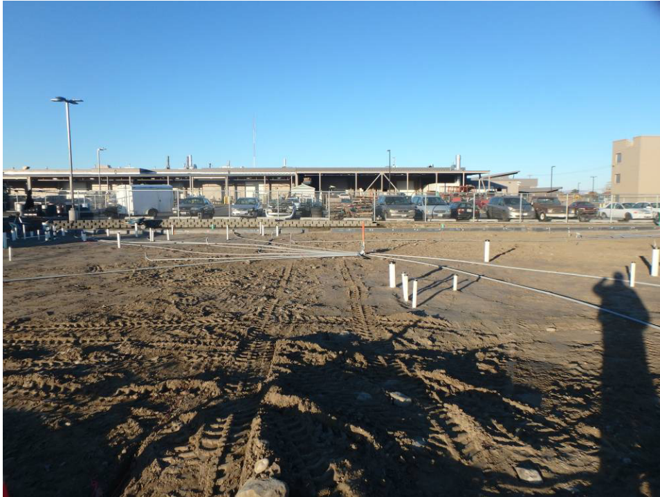
Looking west at the sub-slab conduit
