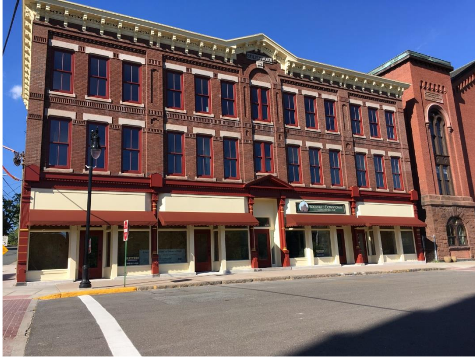
Citizens Block Building, Vernon CT
