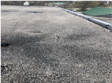
The roof is in good condition
