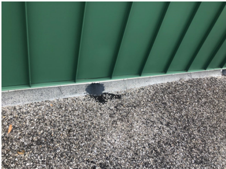
The roof is in good condition
