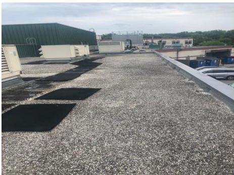
Roof is in fair condition
