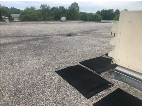
Roof is in fair condition
