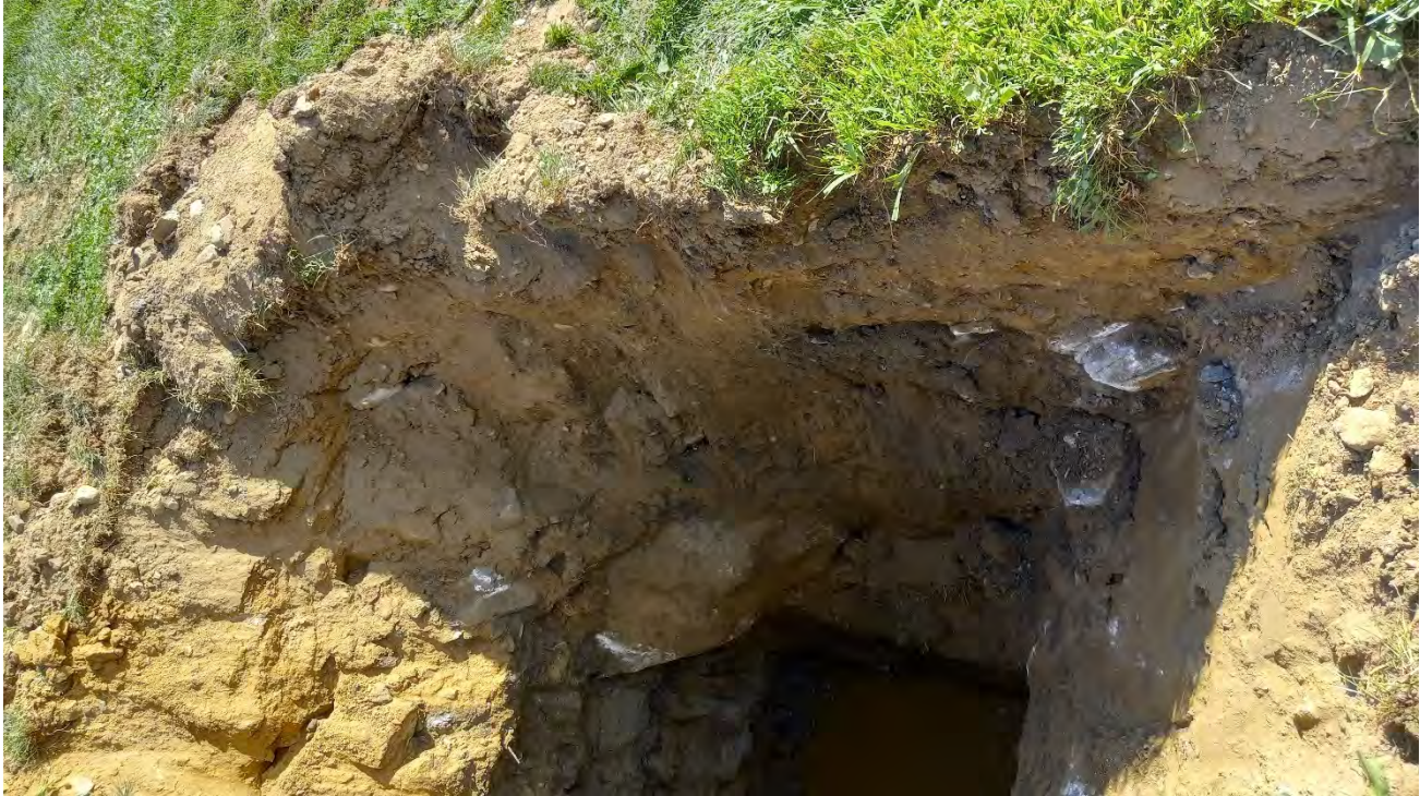
In progress TP-03. – Short-term equilibrium groundwater level measured at approximately 7 feet below ground surfaces
