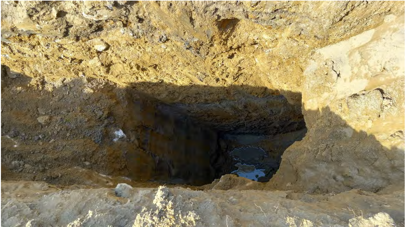
In progress TP-08. – Short-term equilibrium groundwater level measured at approximately 9.0 feet below ground surfaces
