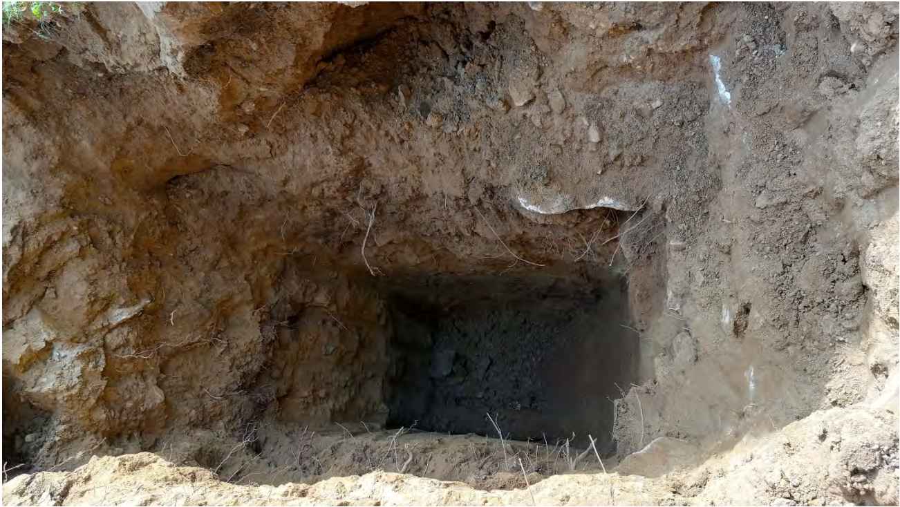
In progress TP-09. – Short-term equilibrium groundwater level measured at approximately 8.5 feet below ground surfaces
