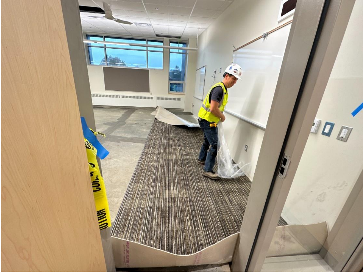
Carpet being installed in one of the general education classrooms
