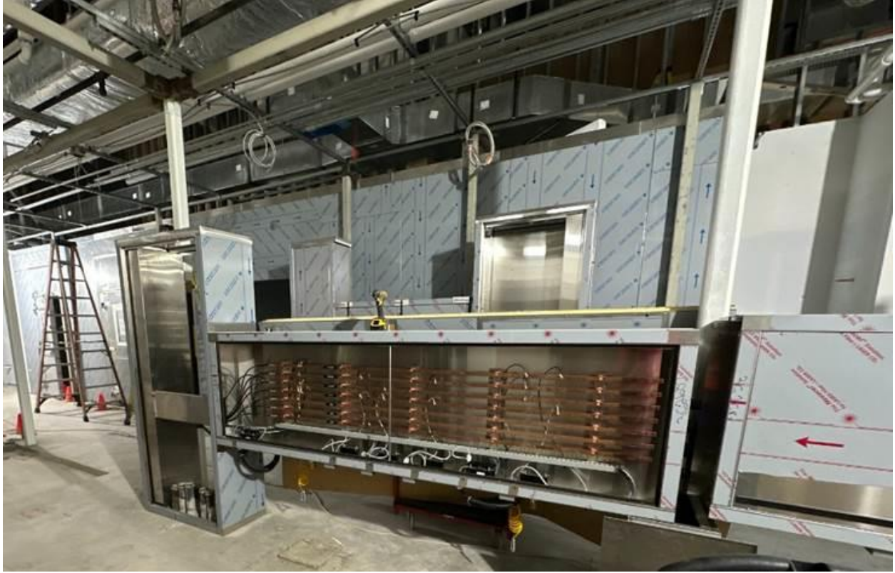
Kitchen line equipment is being installed
