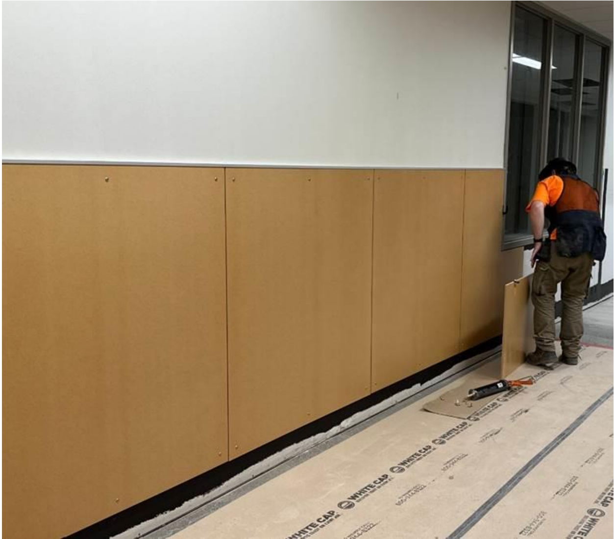
Crews installing wainscoting (decorative wall panels) in Academic Wing
