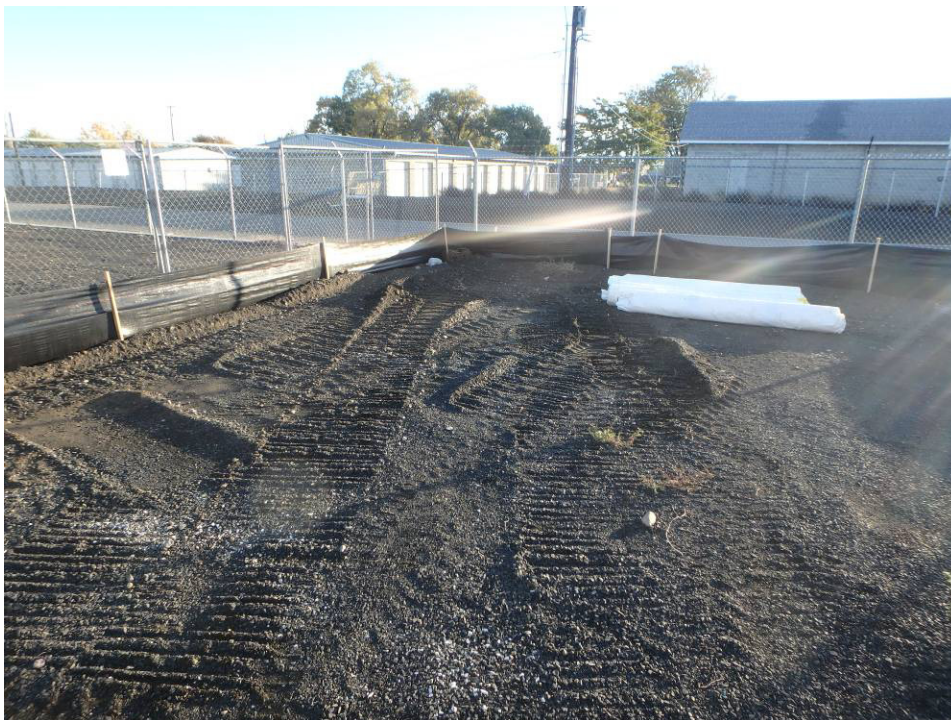
Silt fence at the northeast corner of the site
