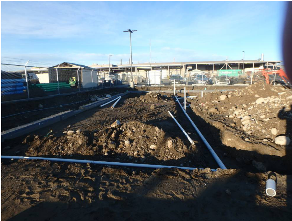
Looking west at the south sub-slab piping
