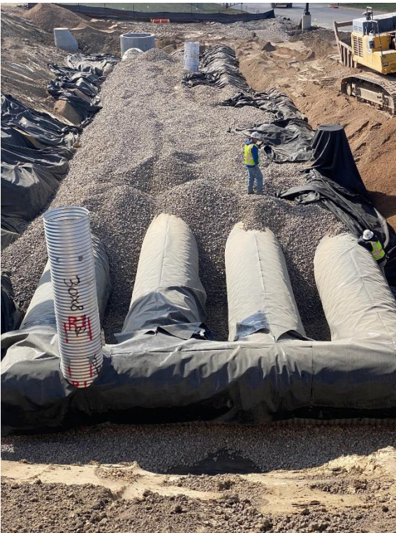
Underground Storage System installed and being backfilled
