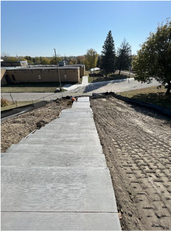
Concrete forms removed and backfilled for stairs
