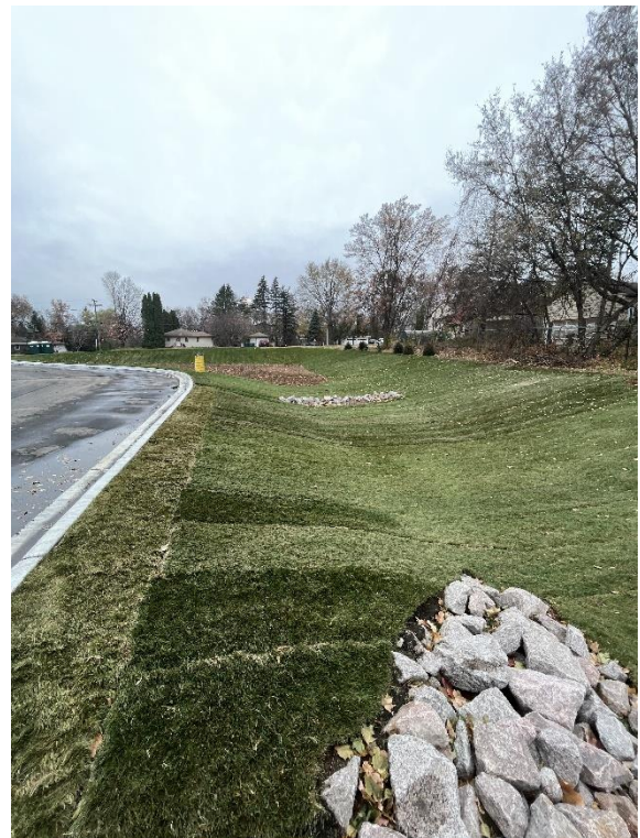
Base course of paving and final landscaping installed
