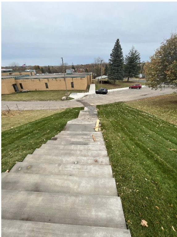
Final landscaping installed
