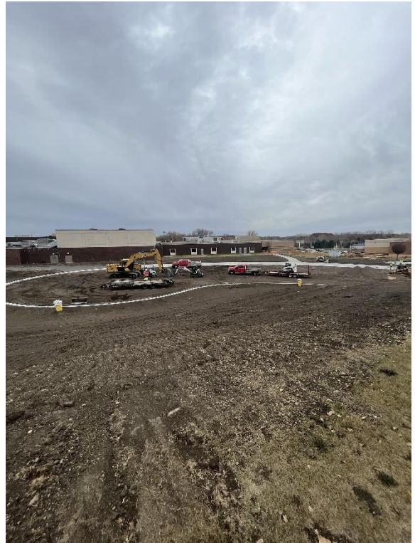
Curbing and sidewalks installed across entire site
