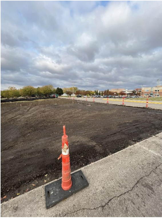
Pavement Removed on South HS Lot and drives
