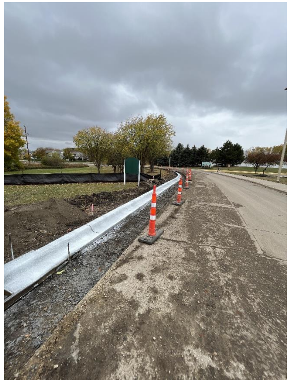
Curbing installed along South HS lot and Drives
