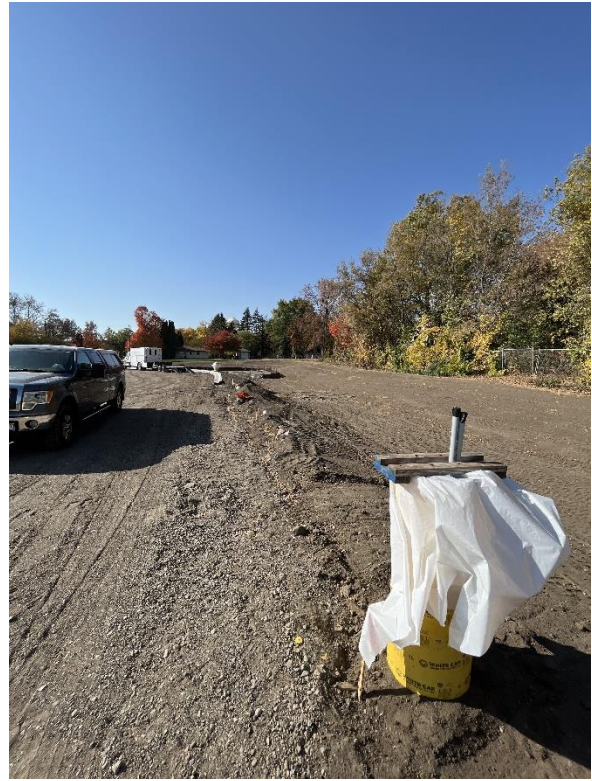
Installed and poured concrete for new light poles
