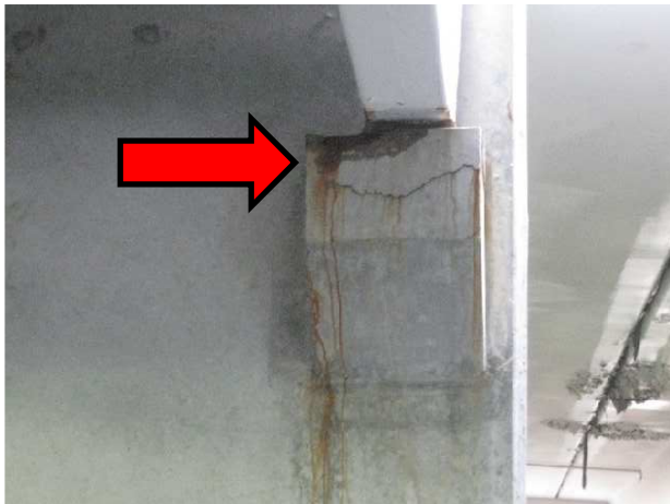
03 Spalled and cracked corbel with corroded embed plate
