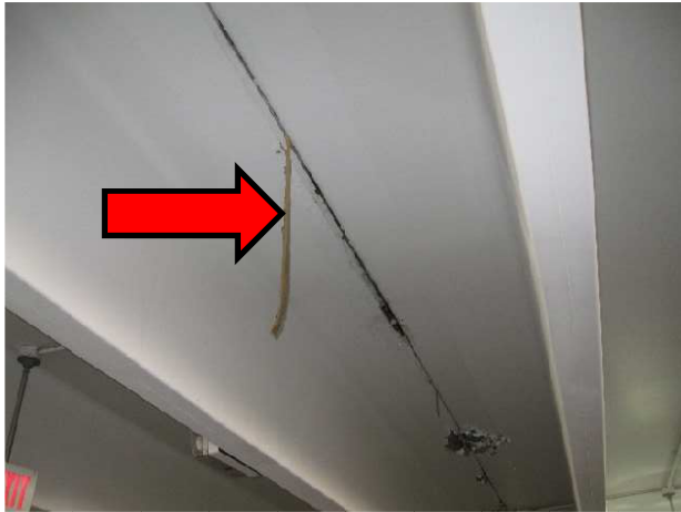
01 Deteriorated sealant at double-T joint
