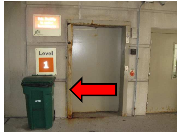
24 Corroded elevator frame
