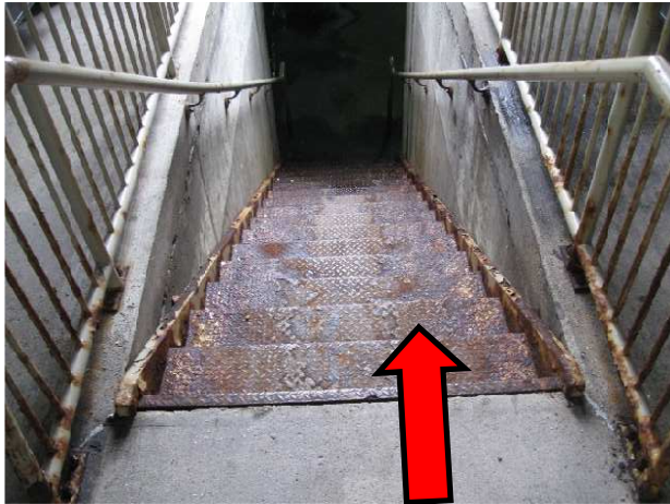
13 Corroded stair treads, stringers and guardrails
