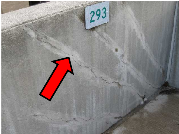
15 45-degree cracks at spandrel panel
