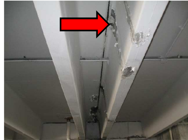
02 Water damage and peeled paint
