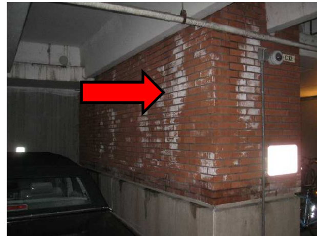
28 Efflorescence at brick facade
