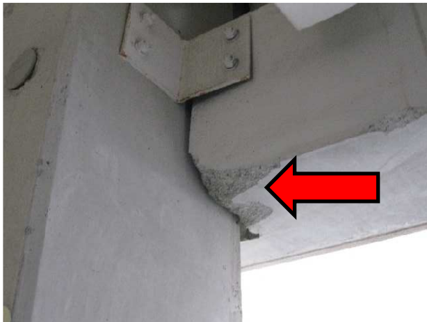
07 Spalled concrete at underside of beam
