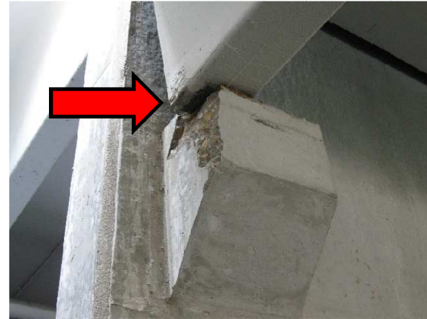
04 Double-T partial bearing at corbel
