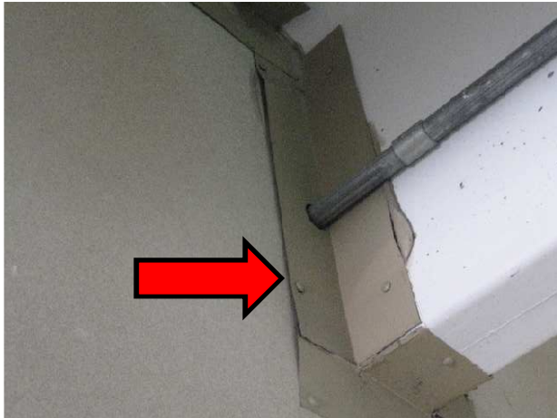
29 Flashing with no sealant at beam penetration
