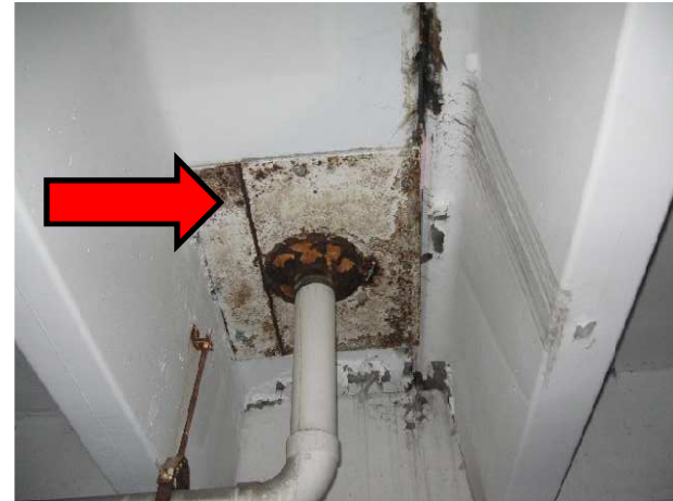
26 Corroded plate at drain
