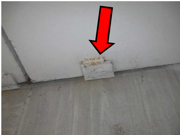
11 Corroded shelf angle
