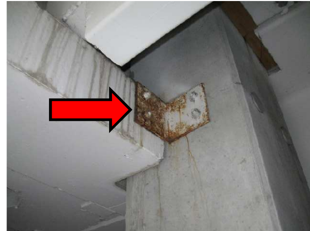
10 Corroded steel angles at beam-to- column connection
