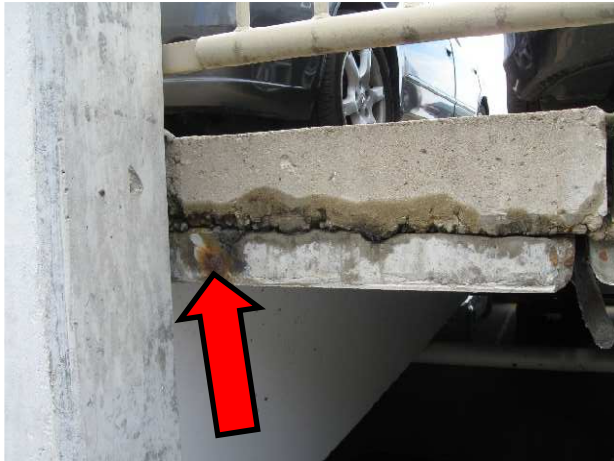
17 Exposed corroded rebar at precast double-T beam flange
