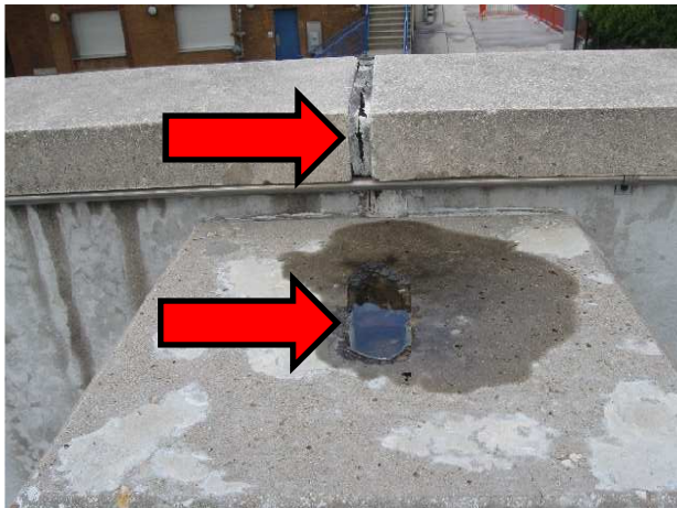
19 Spalled concrete and open sealant joint at coping
