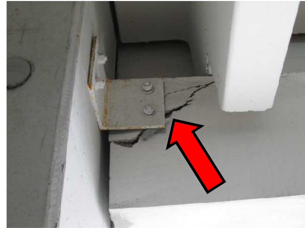
06 Spalled and cracked concrete at beam anchor point
