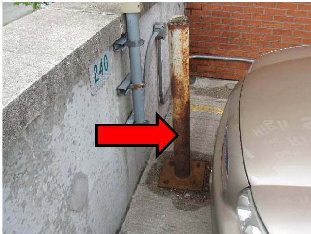
23 Corroded bollard
