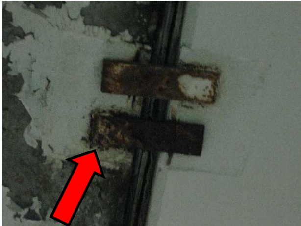
09 Corroded connector plates at expansion joint
