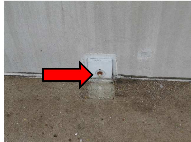
22 Corroded anchor bolt
