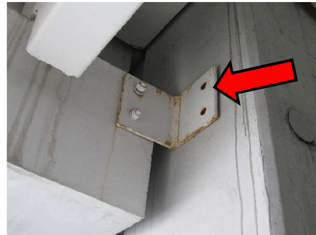
12 Corroded steel angle with missing anchor bolts
