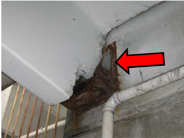
05 Corroded steel saddle
