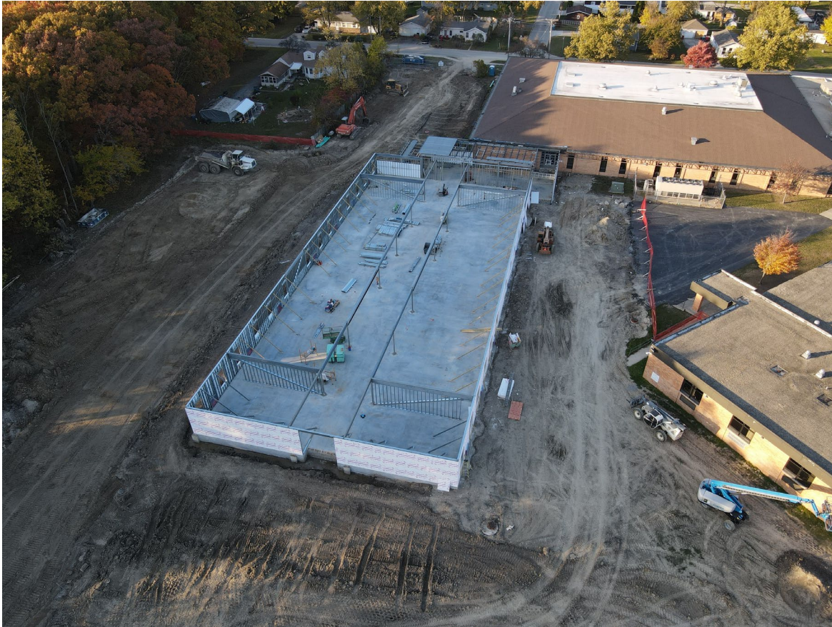
Classroom Addition Exterior Framing
