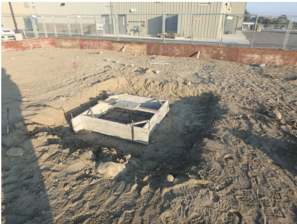
Formwork for the north pad footing
