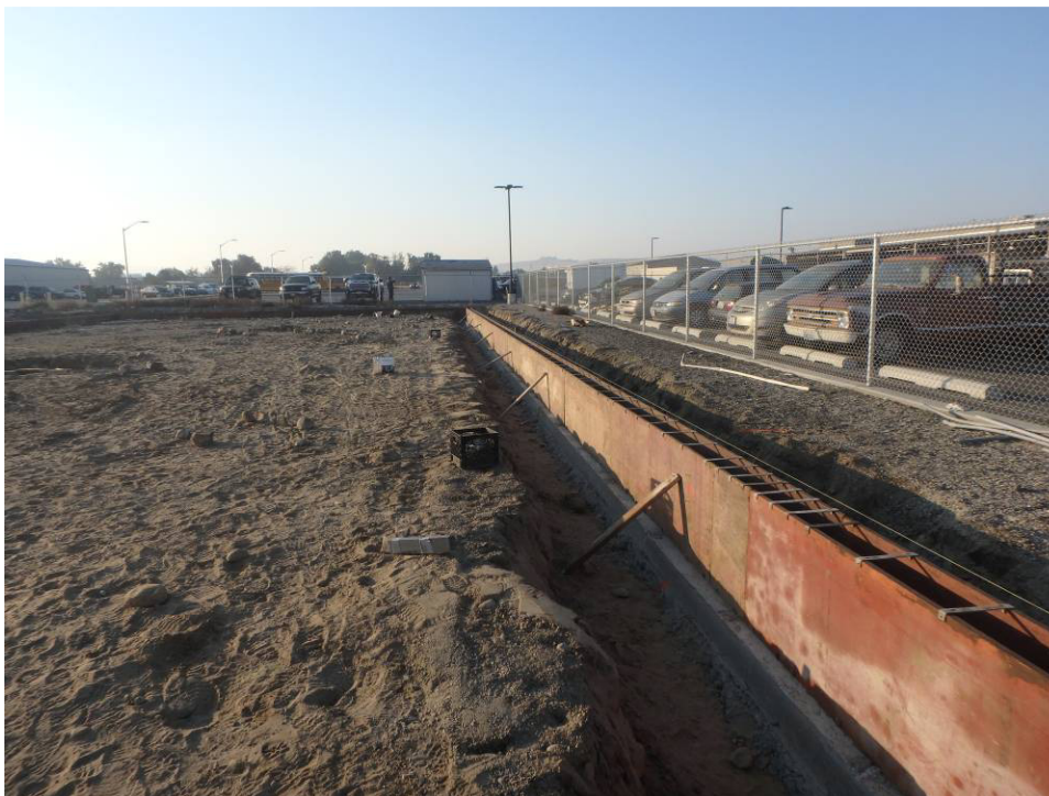
Looking south at the west foundation wall forms
