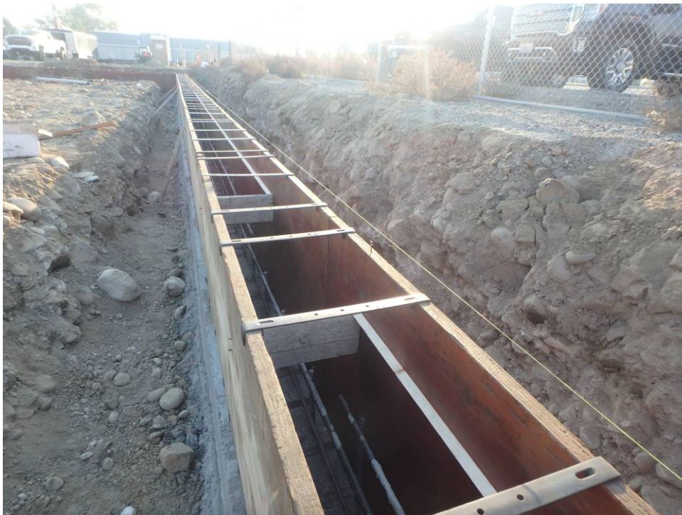
Looking east at the south trench and foundation formwork
