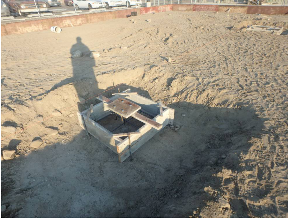
Formwork for the center pad
