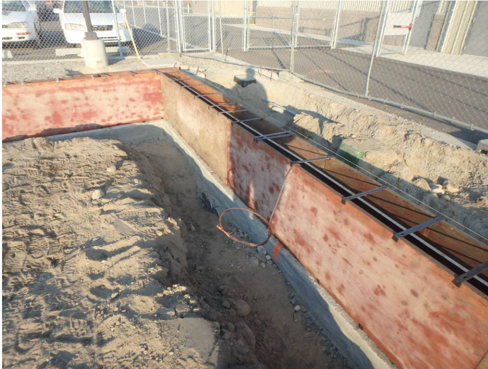
Northwest corner of the building foundation wall formwork and sleeves
