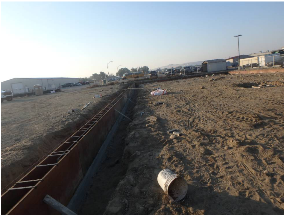
Looking south at the east foundation wall forms
