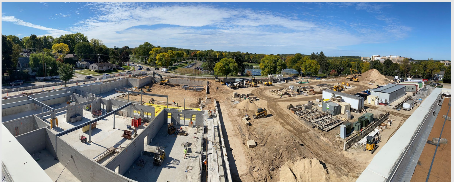
In the new pool and gym addition, CMU walls and structural steel are installed in preparation for concrete slabs coming later this month
