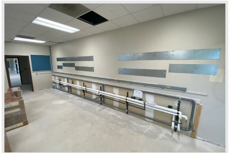
Work continues in renovated science lab spaces where walls are being prepped for new casework
