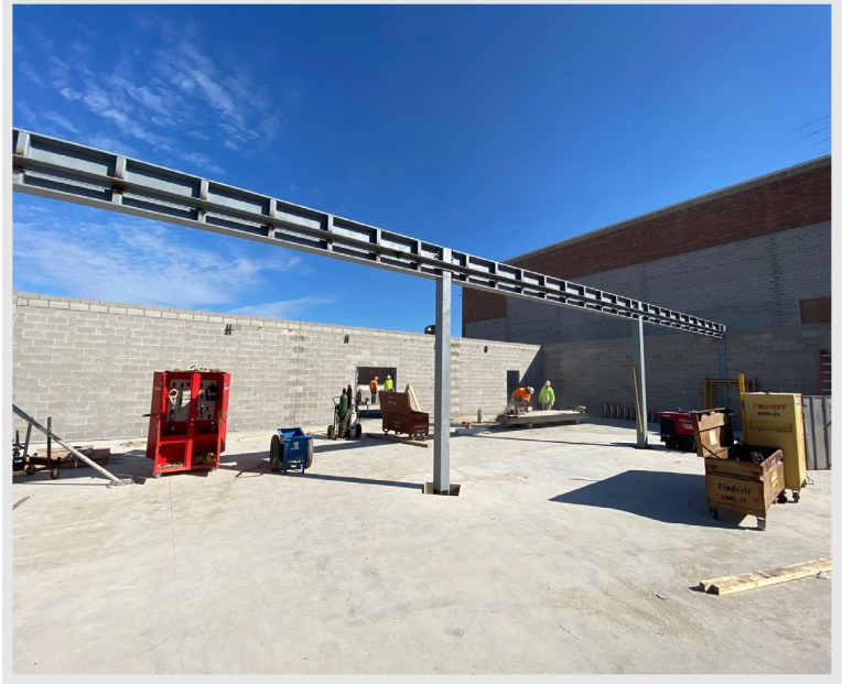
Structural steel was recently installed in the future weight room area, which will support the second floor of this new addition
