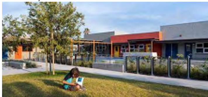
Elementary School with window upgrades. Similar materials to be used for Limerick ES upgrades
