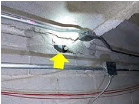
Roof-Wall Intersection Air Sealing – the exterior flashing and finishes at the roof-wall intersection are not constructed to stop air leakage (Upper Providence ES).
