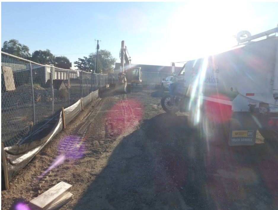
Looking east along the southeast project site
