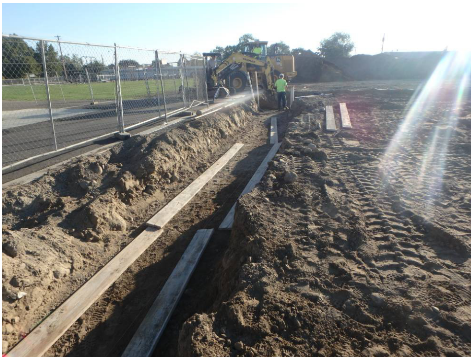
Looking east along the north foundation trench
