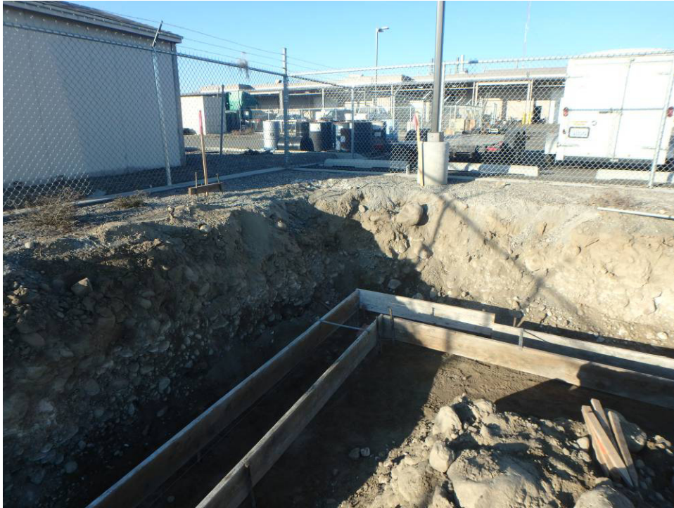
Southwest corner of the building footing trench
