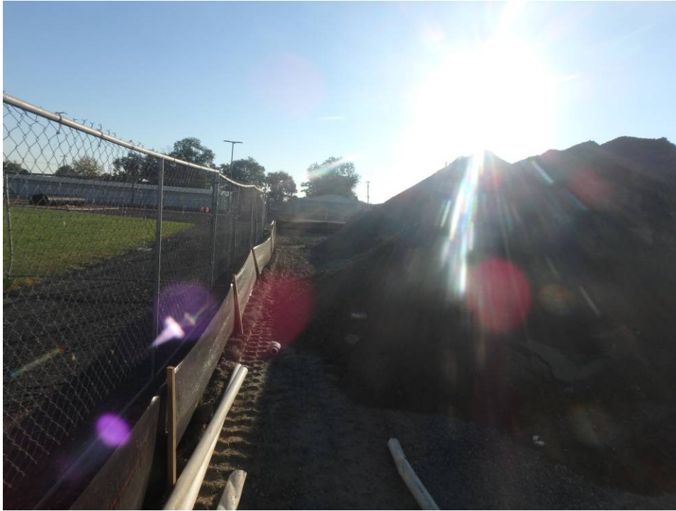
Looking east along the north project site to the northeast corner
