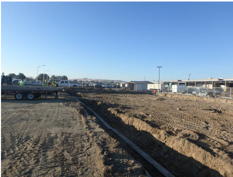
Looking south at the east foundation wall trench
