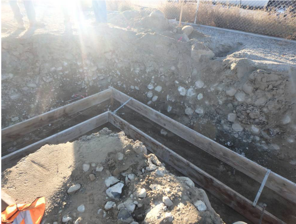
Southeast corner of the building footing trench
