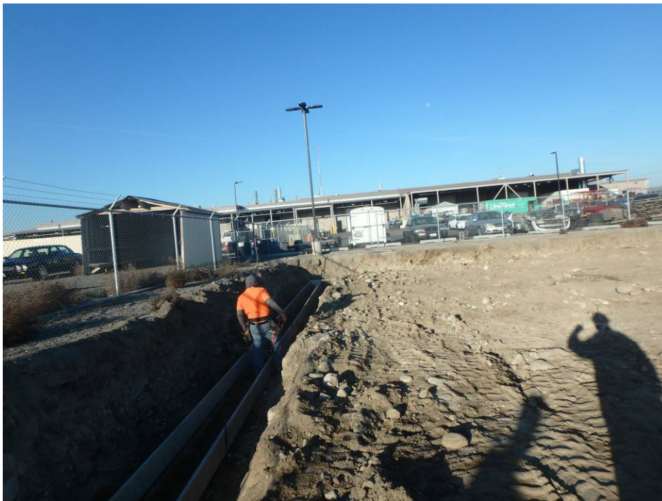
Looking west across the south trench and footing formwork of the building
