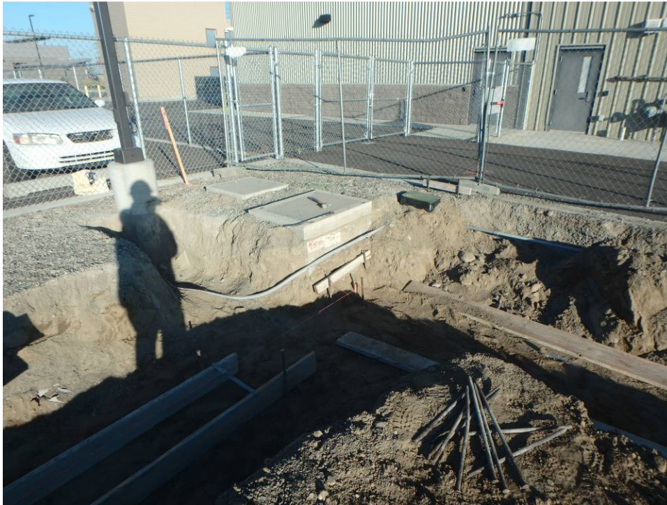
Northwest corner of the building footing trench looking west
