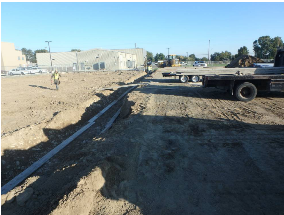
Looking north across the east side of the building footprint
