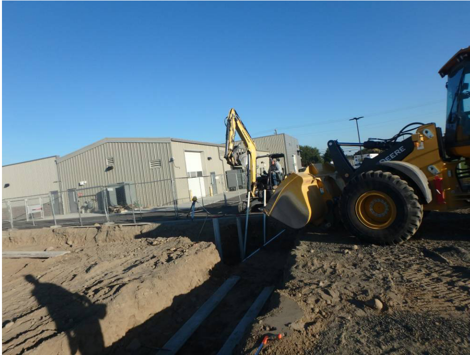
Forming the thrust block
