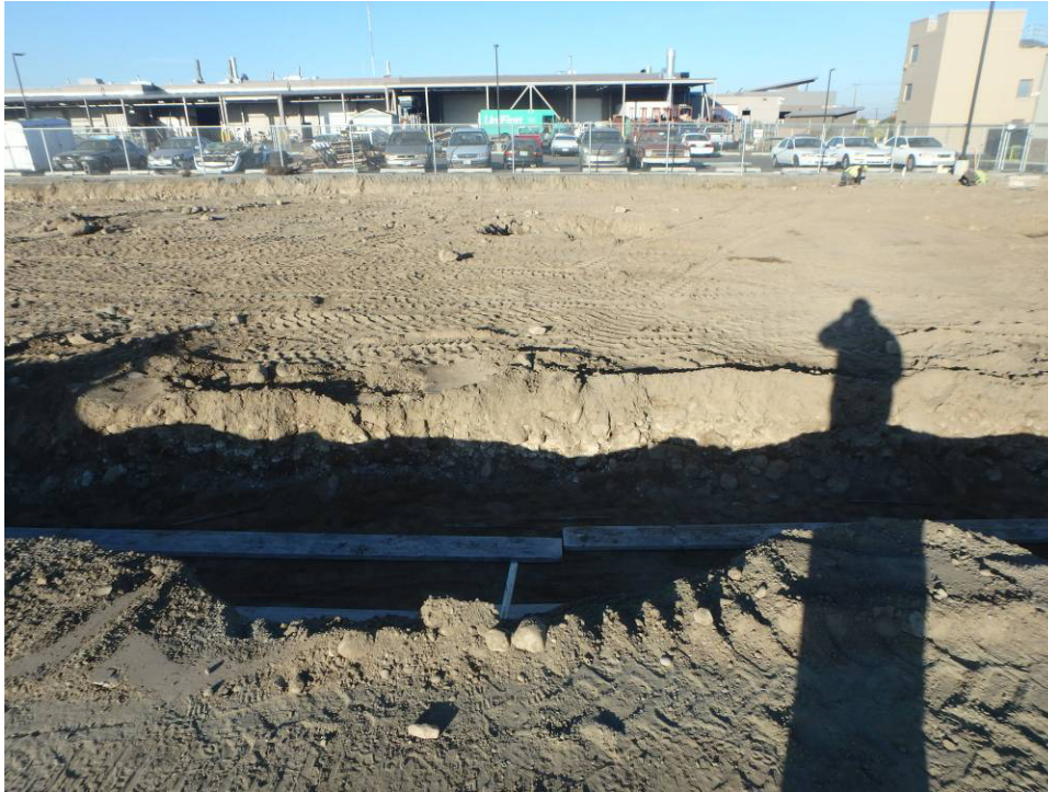
Looking west across the center of the building footprint
