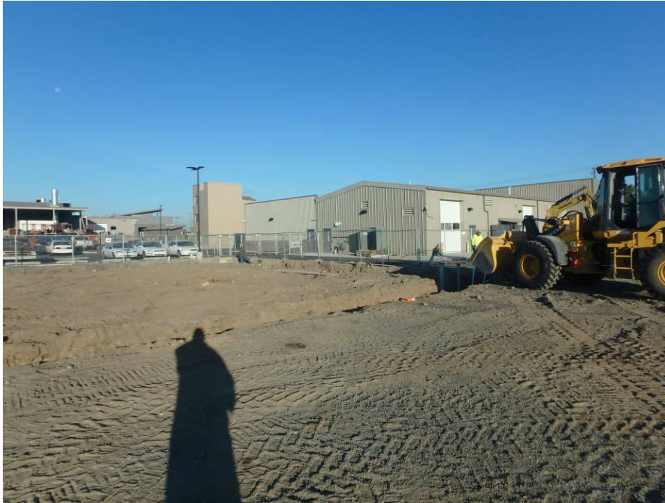
Looking at the northeast corner of the building footprint
