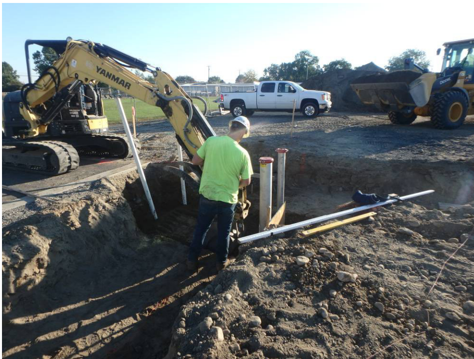
Base rock for the thrust block
