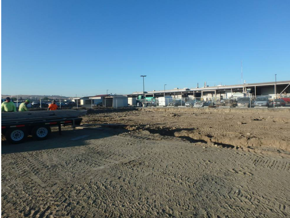
Looking southwest across the building footprint
