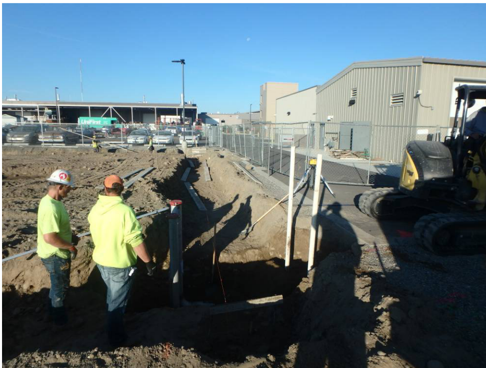
Looking west along the north foundation trench
