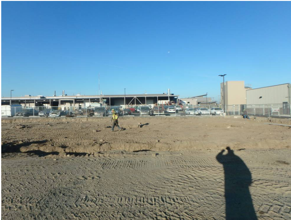
Looking west at the north half of the building footprint and
