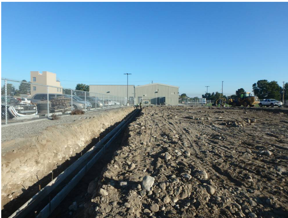
Looking south at the west foundation wall trench
