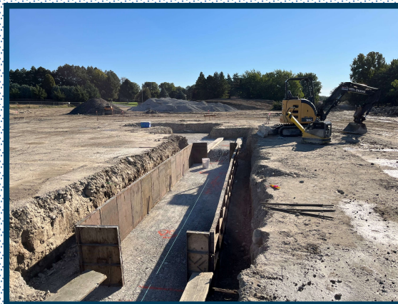
Footing Excavation & Forming Ongoing
