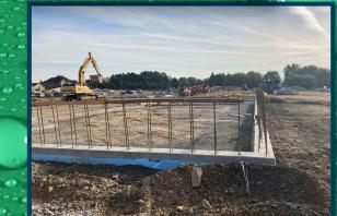
B-1 Foundation Backfill & CMU Block Layout
