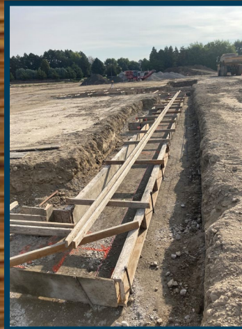
Footing Formwork in Progress
