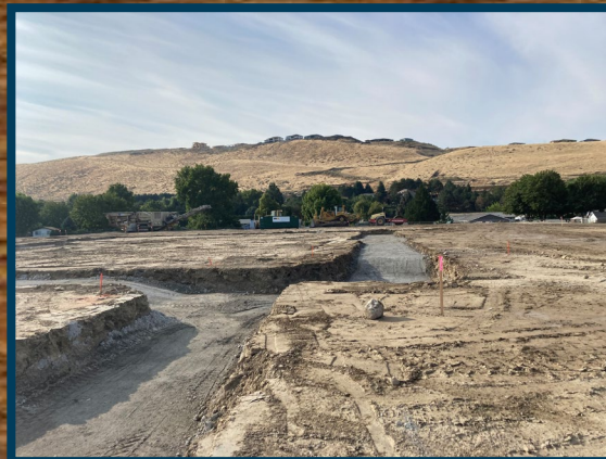
Footing Excavation & Fill
