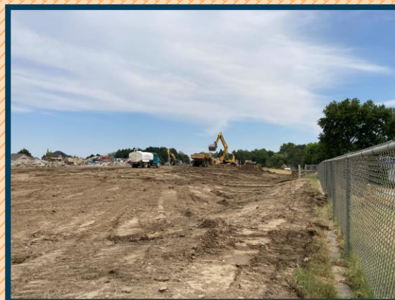
Sitework Clearing & Demo
