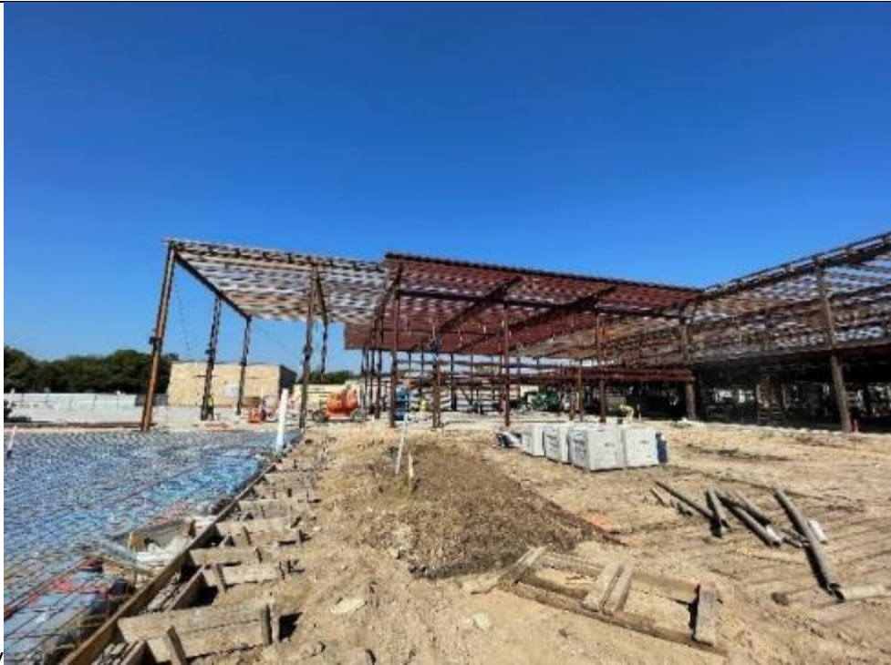
Structural steel area B
