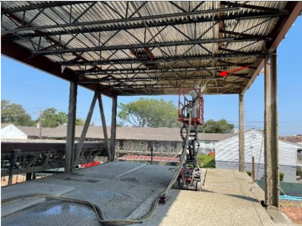
Structural fire proofing area C
