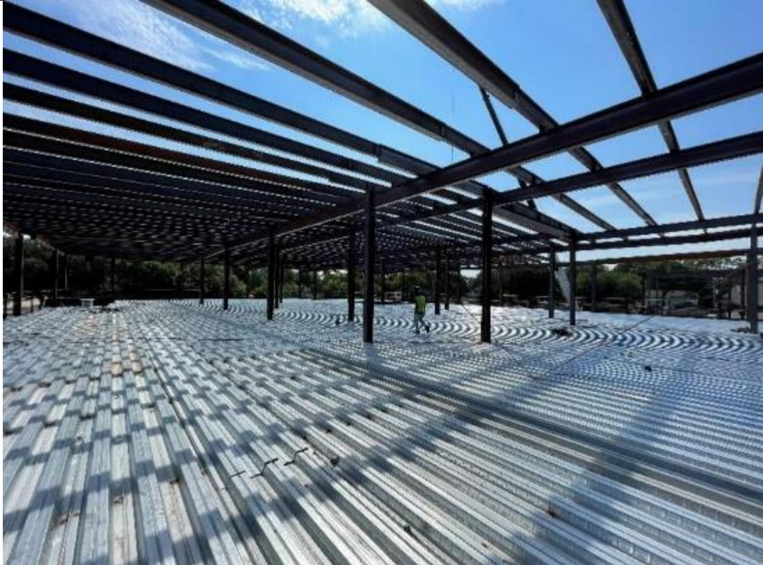
Metal Deck area C
