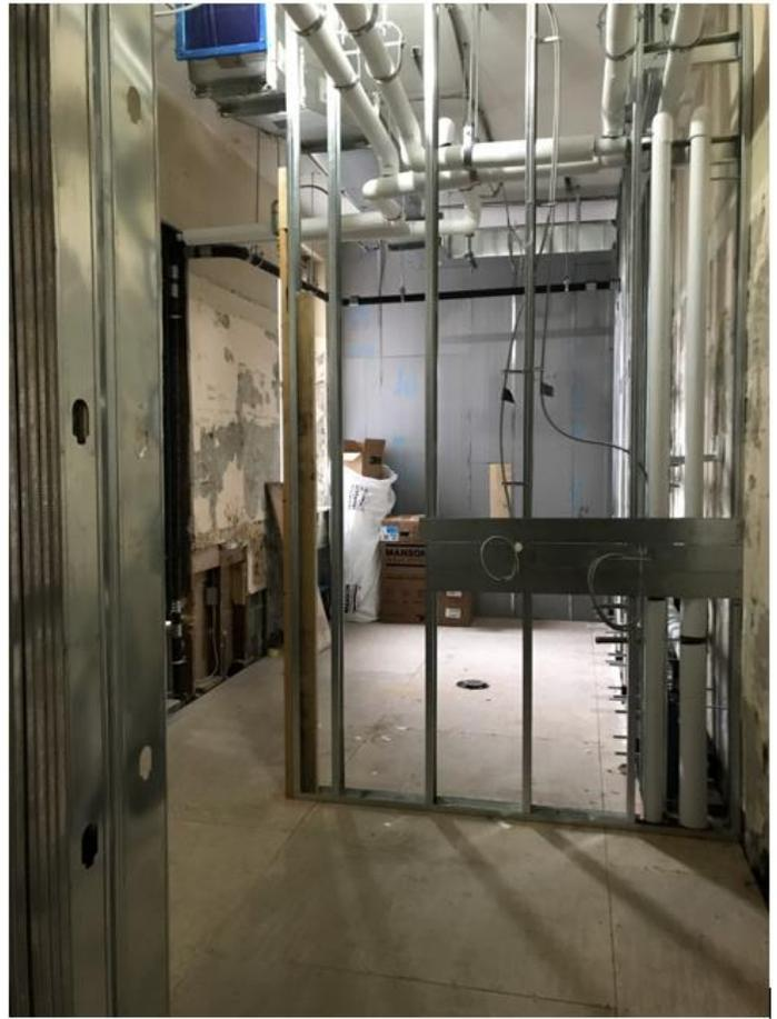
**Our bathroom walls are being framed and all new pipework is being installed.**
