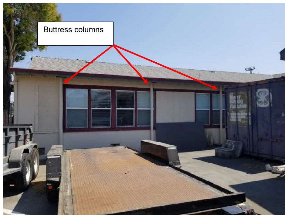
Figure 9 – Building 400 buttress columns
