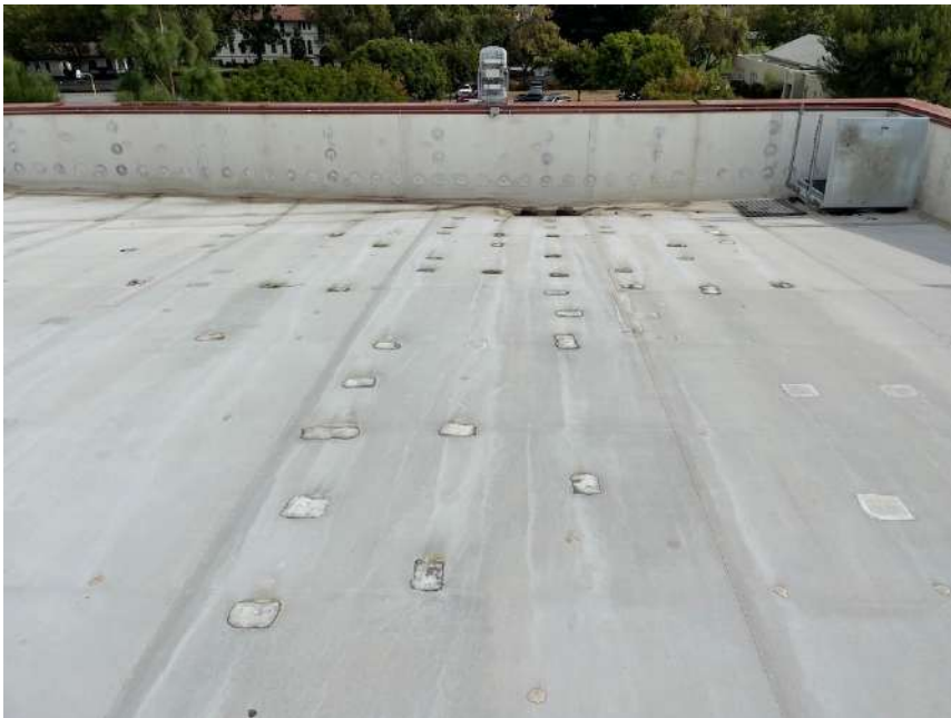
Previous patching made to address this condition.
