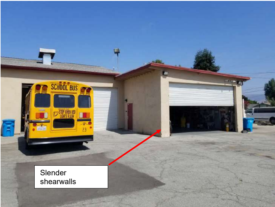
Figure 8 – Building 100 eastern shearwalls
