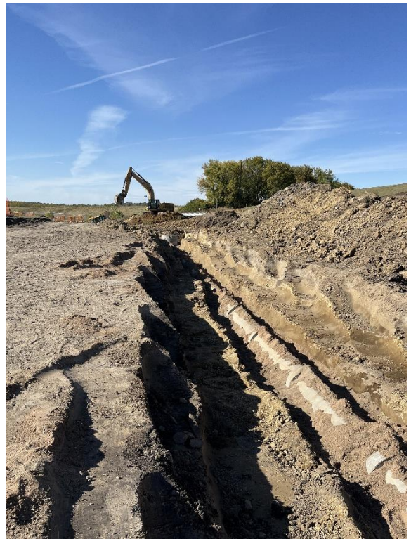
Storm sewer pipe installation in progress
