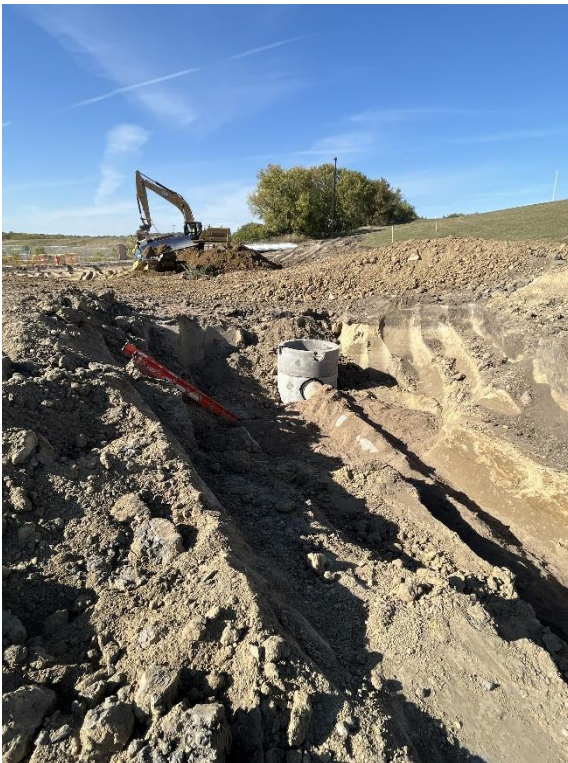
Storm sewer structure installation in progress
