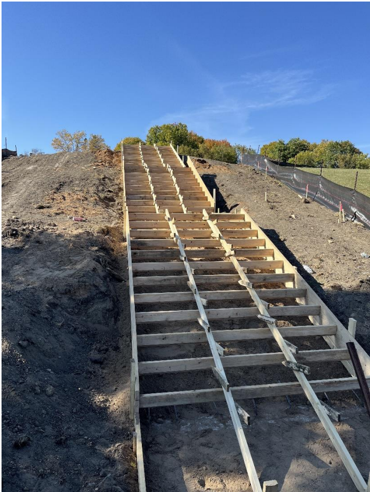
Forms for concrete stairs installed leading to North entry of MS
