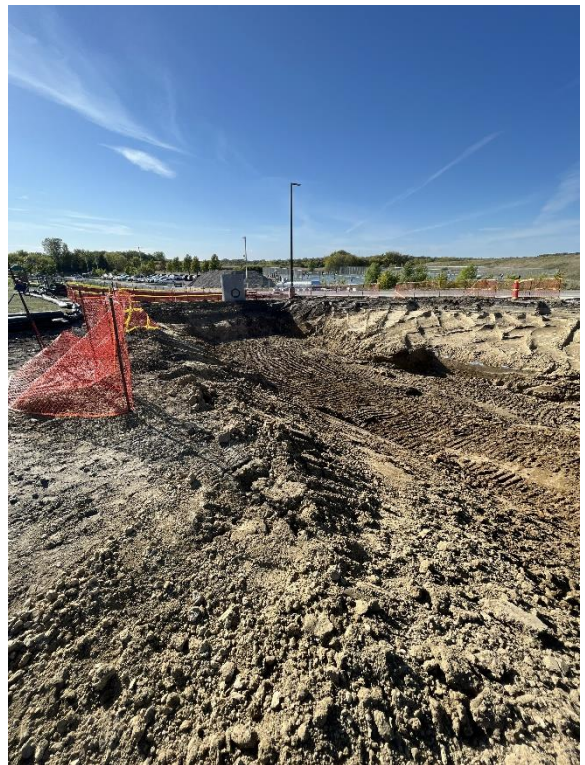
Excavation for underground storage system in progress, with average depths of 20'
