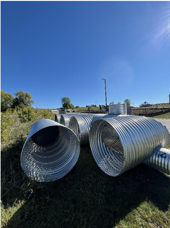
Underground storage system arrived on site and staged for installation
